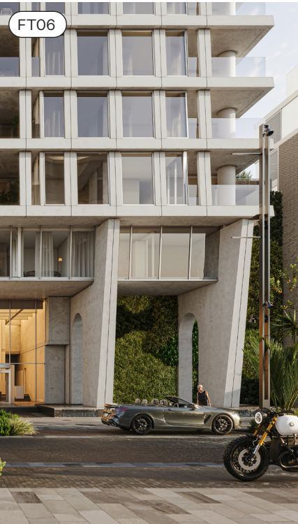
Exposed Concrete at The Base
