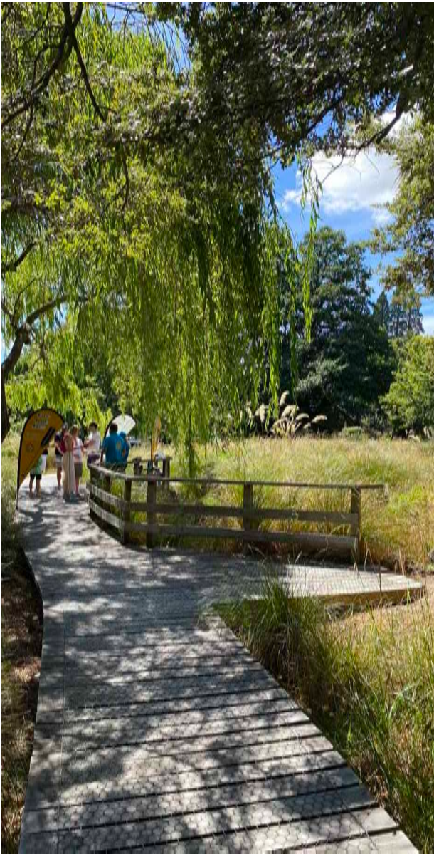
Typical example boardwalk
