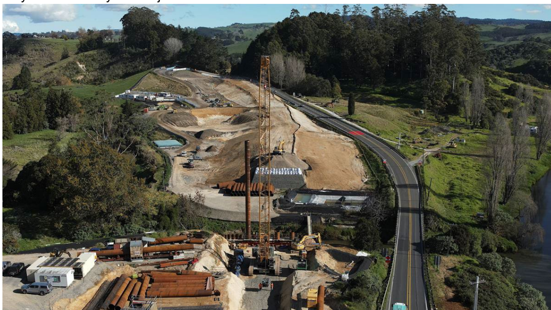
Figure 5 – Extract from SH29 Ōmanawa Bridge Replacement – Site Works Newsletter Photography- December 2025 8
