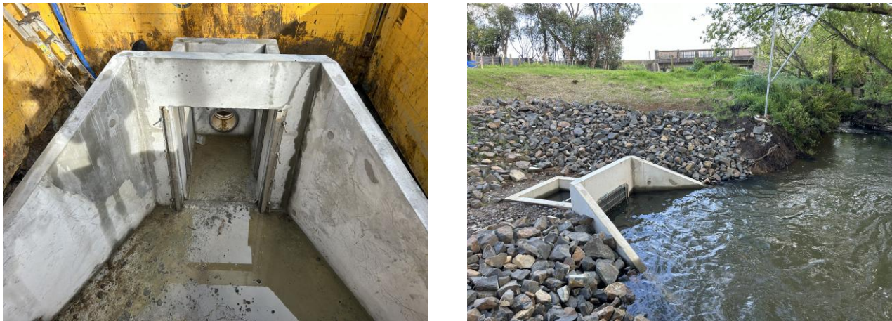
Figure 3. Examples of wingwall arrangement and installation. a) precast wingwall, and b) wingwall installation in stream channel showing grate.
