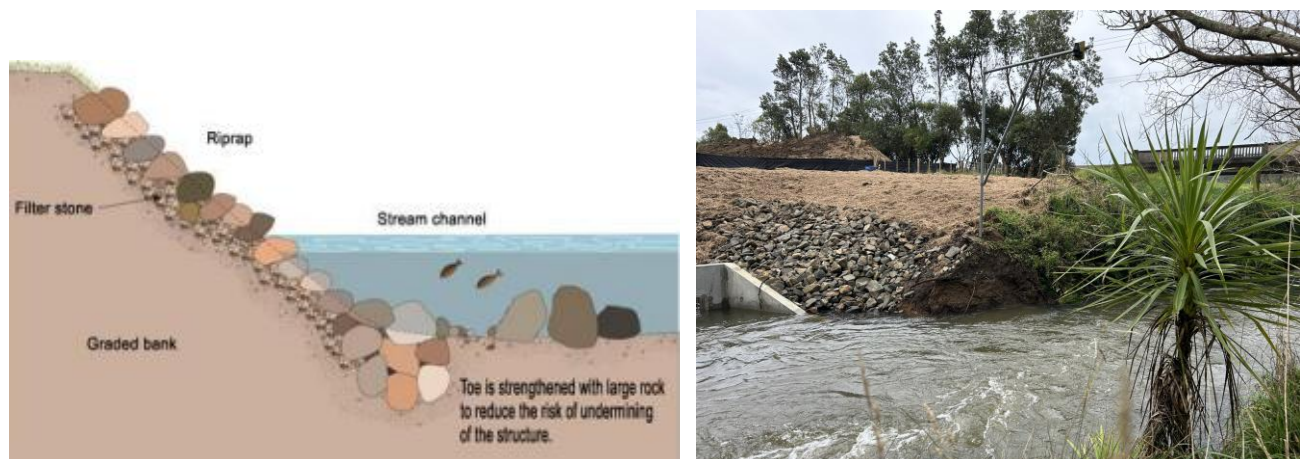
Figure 4. Examples of stream bank armouring using rip rap. The right photo shows the stream intake at Muriwai.
