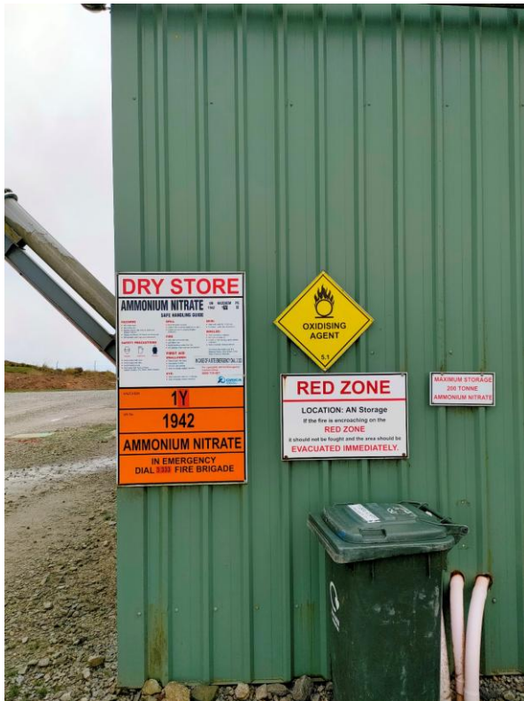
Figure 6.1: Signage signalling oxidising substance hazard at the AN prill storage building within the Class 5 explosives mixing and preparation compound.
