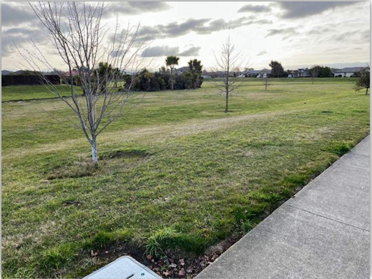
Figure 4-19: Example of a stormwater attenuation basin in Rangiora showing gradients and grass coverage.
