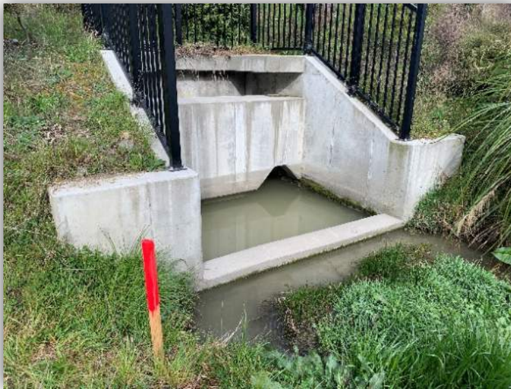
Figure 4-22: Example of an energy dissipation impact basin and riprap apron to minimise erosion
