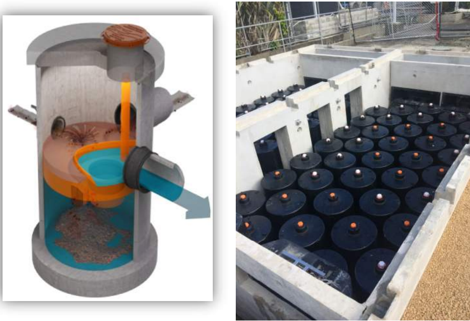
Figure 4-18: (Left) Typical proprietary GPT manhole as Stage 1 treatment. (Right) Proprietary filter.
