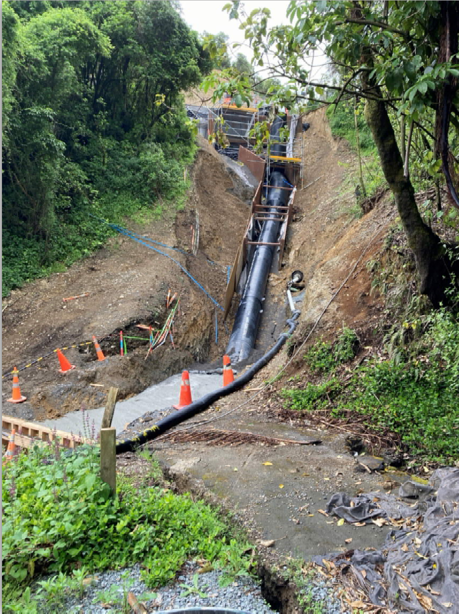
Figure 4-21: Example of a steep polyethylene pipeline down a low strength bank, to an energy dissipation impact basin, Culvert 880, SH58, Wellington
