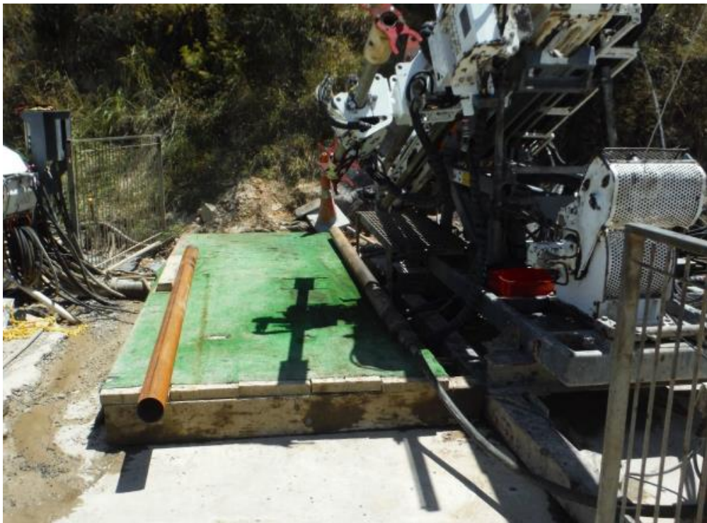
Figure 33: Drill rig with wooden platform
