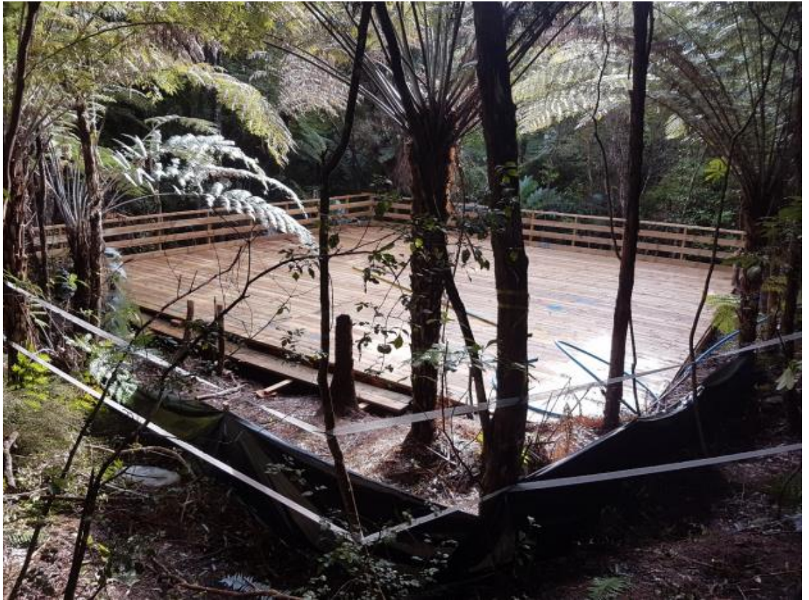
Figure 18: Typical exploration drill site with raised wooden drill platform.
