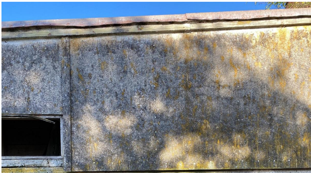
Figure 5.11: Shed with fibre cement cladding.
