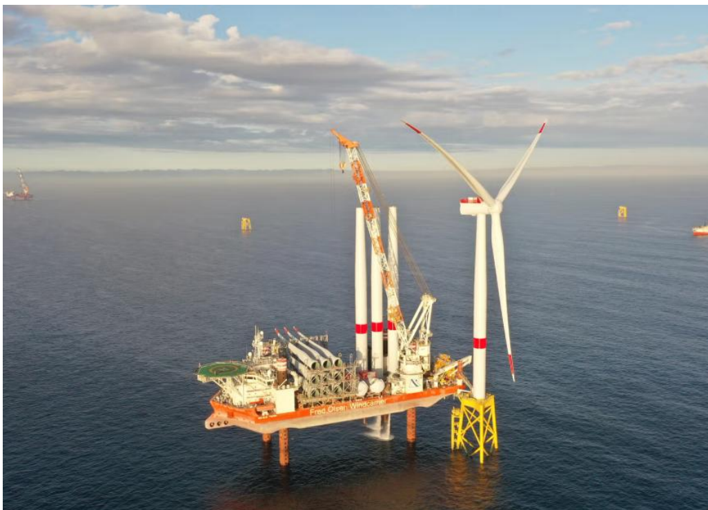
Figure 1: A Jack-up vessel constructing an offshore wind turbine generator.
