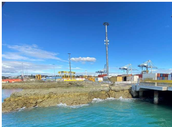
Photo 7 – Reclamation bund with rock revetment (looking south)
