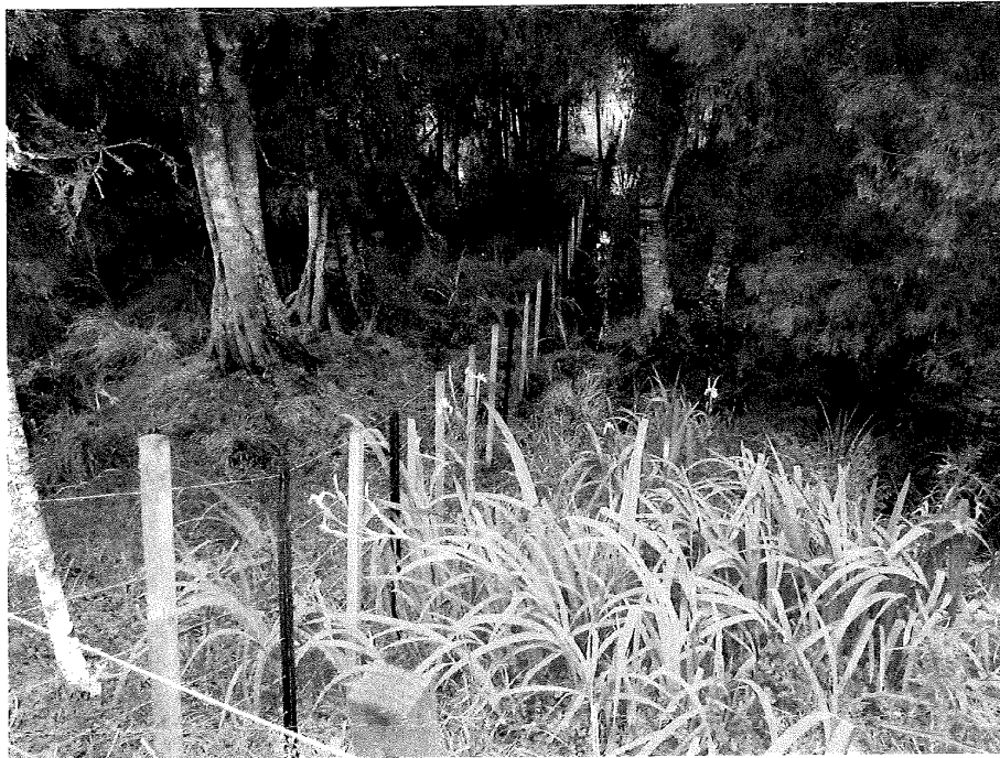
Difficult ground conditions have challenged fencing in places but fences meet or exceed Council's requirements.
