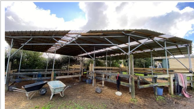
Photograph 13. View of the covered yards, facing northeast.
