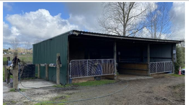
Photograph 14. View of the barn and stables (green building) and the horse washbay (concrete pad to left of image), facing southwest.
