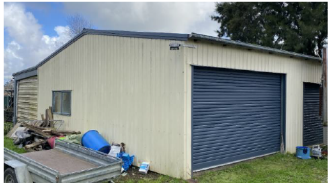
Photograph 12. View of the shed, facing southwest.
