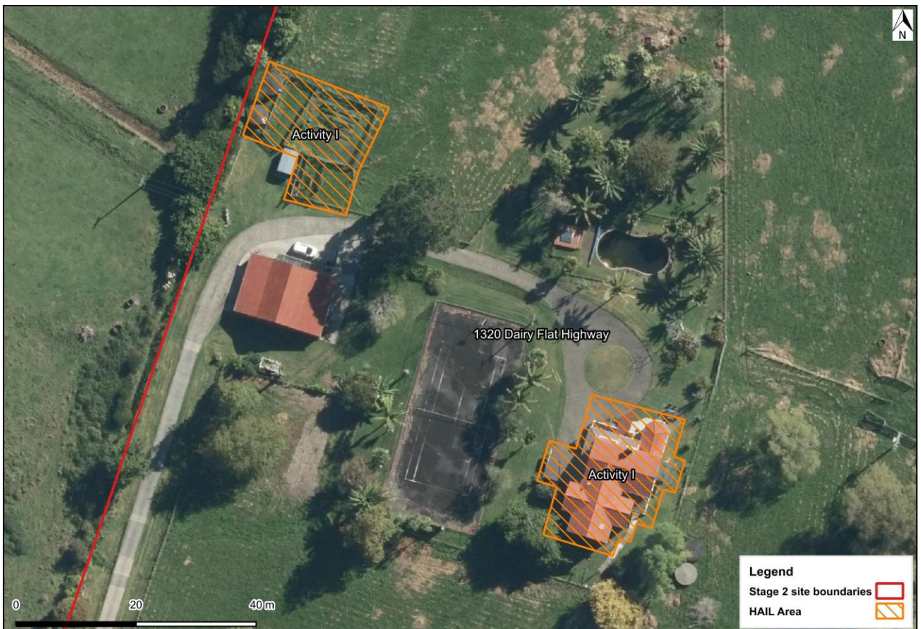
Figure 8. Location and extent of HAIL Activity I on the site (source: LINZ 2024-2025).
