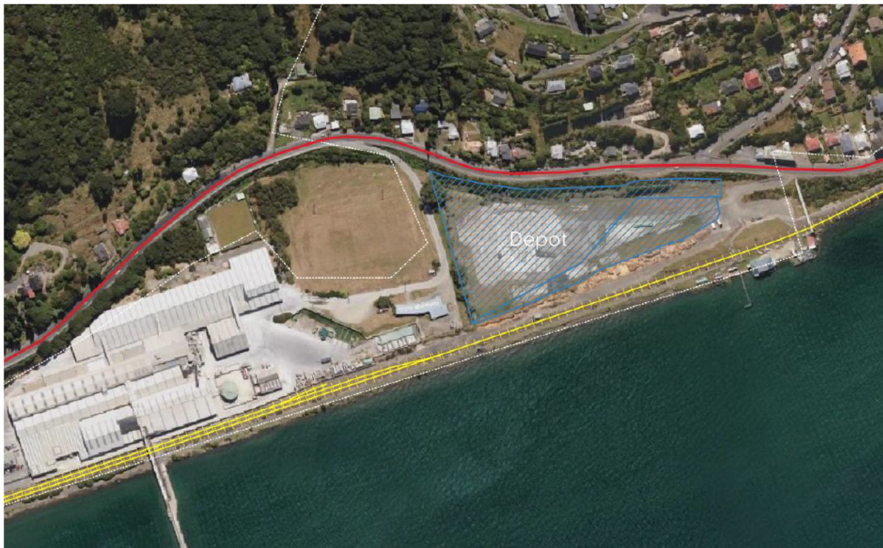
Figure 3.9 – Aerial Image of the Ravensbourne Container Depot
