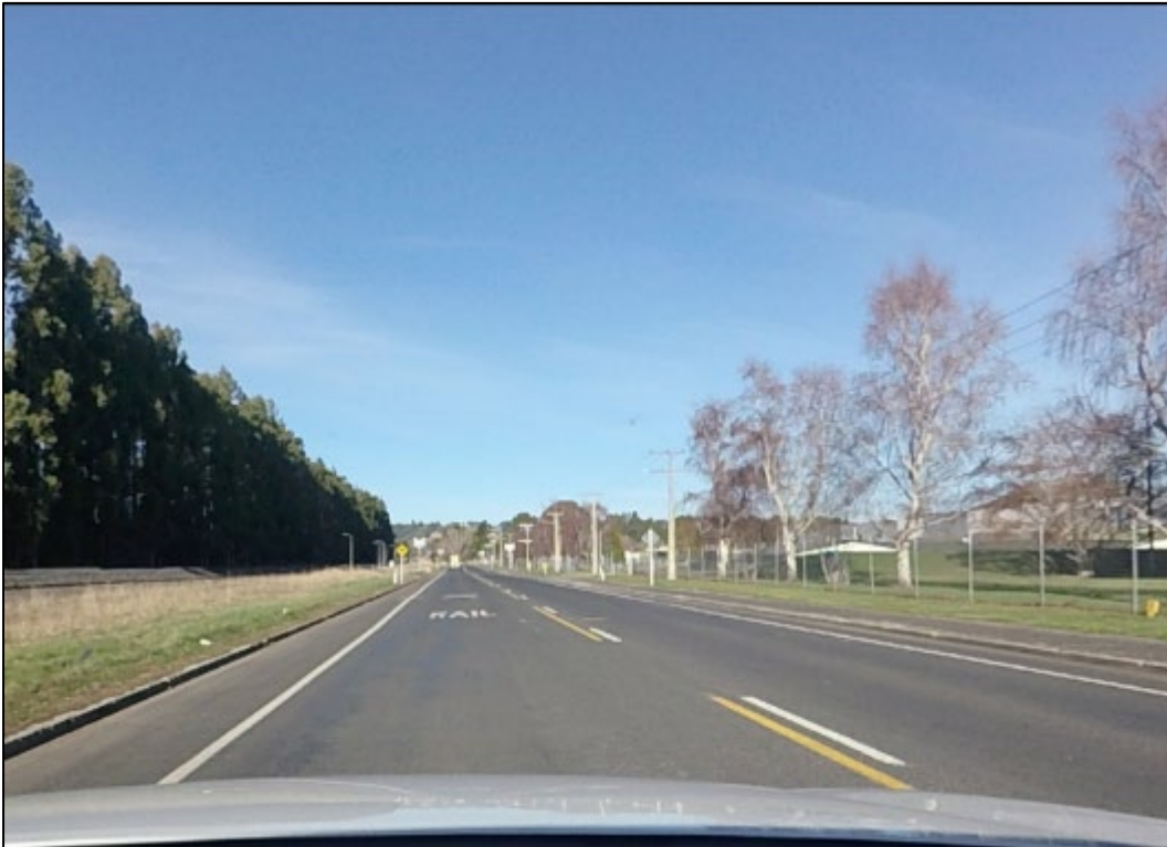
Photograph 3-3: Stedman Road south of Dukes Road North
