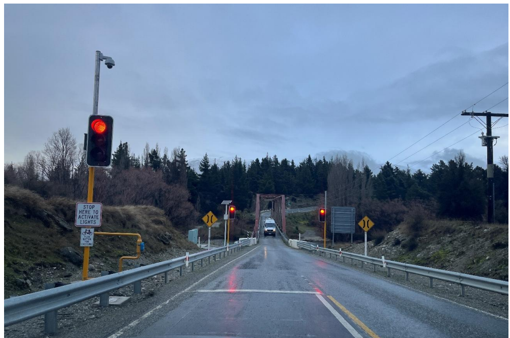
Figure 1: SH8A Red Bridge
