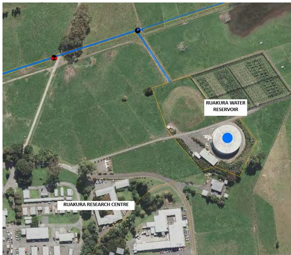
Figure 24 – Ruakura Water Reservoir
