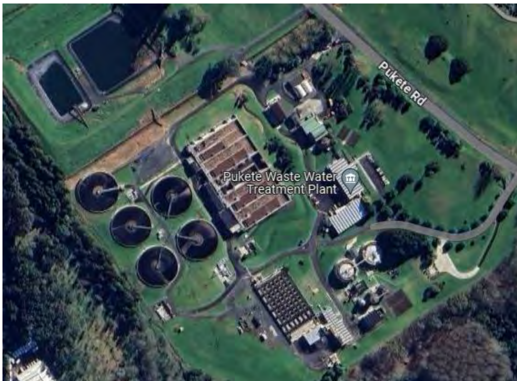
Figure 16 - Pukete Wastewater Treatment Plant (Google Map)
