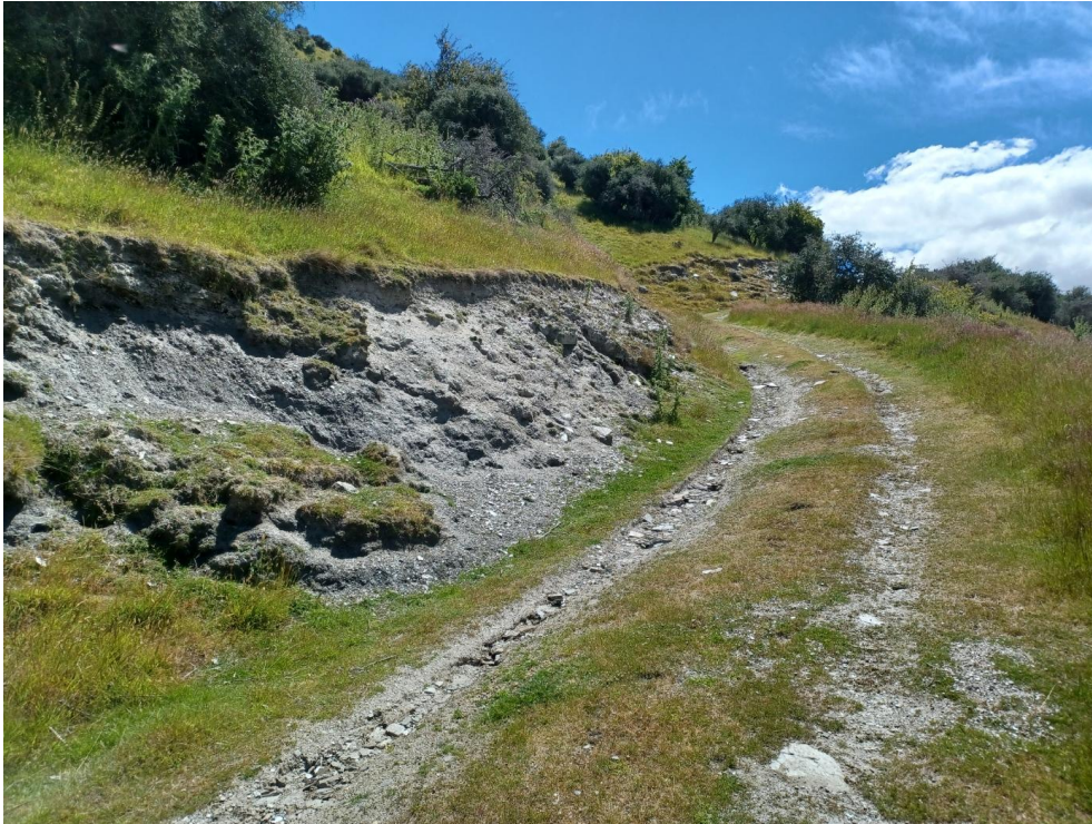
Photograph 2: Overburden soil profiles exposed within the road batters.
