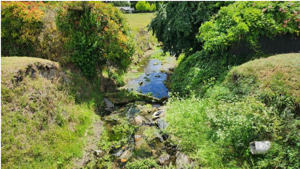
View of From Middle Road
