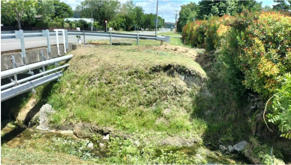
Looking North, Te Aute Road Bridge
