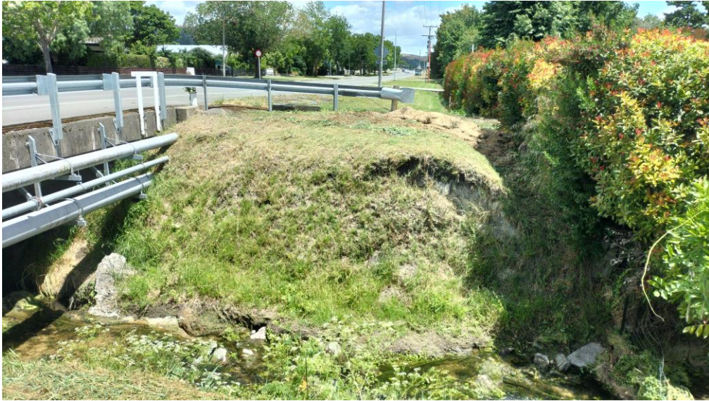
Herehere Stream & Te Aute Road Bridge
