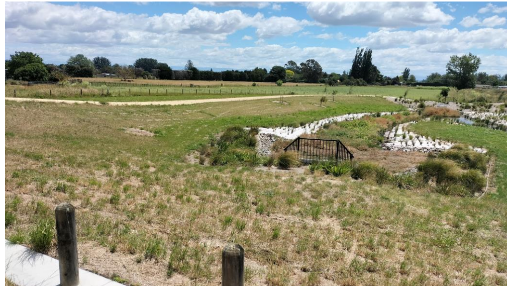
Iona Stormwater Device
