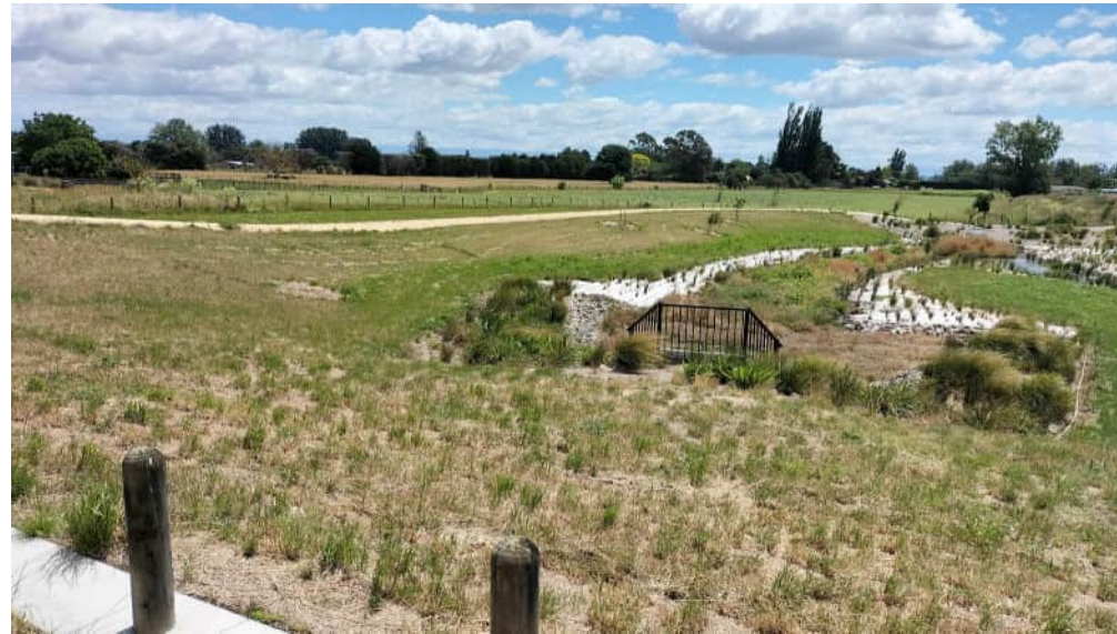
Iona Stormwater Device
