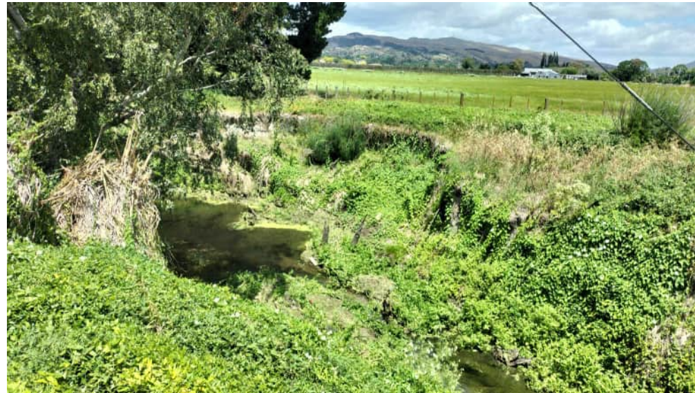
Looking South, Te Aute Road Bridge
