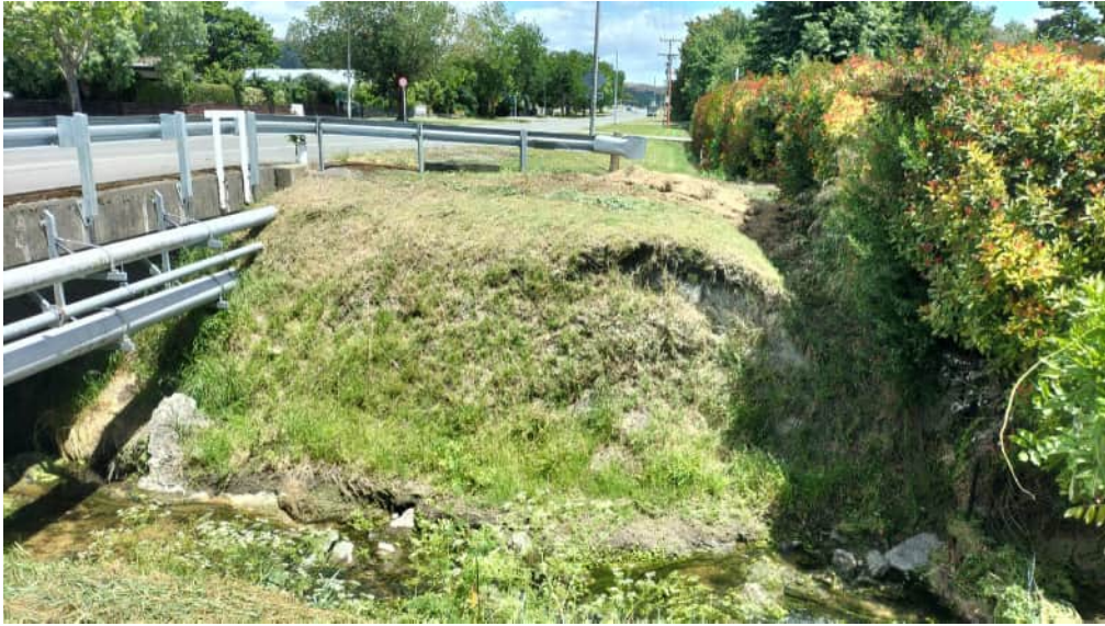
Herehere Stream & Te Aute Road Bridge
