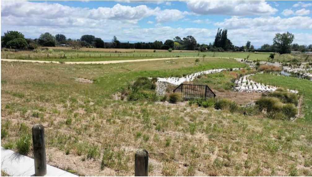
Iona Stormwater Device
