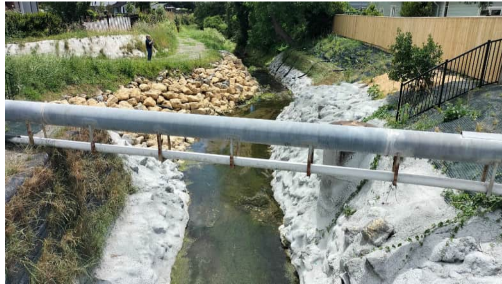
Herehere Stream North of Te Aute Road Bridge
