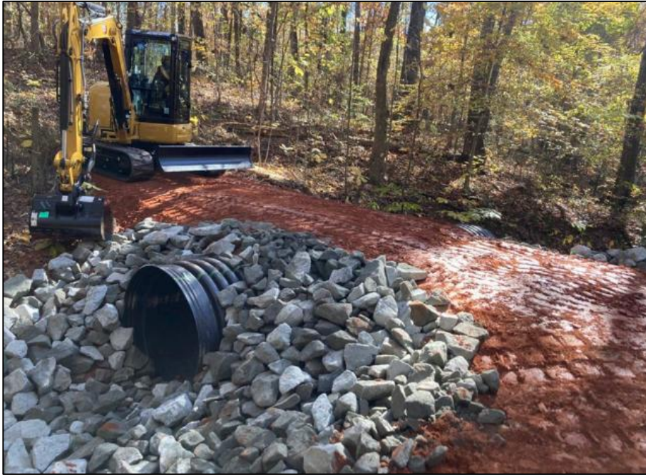
Figure 3-26: Culvert example (Stantec, 2026d).
