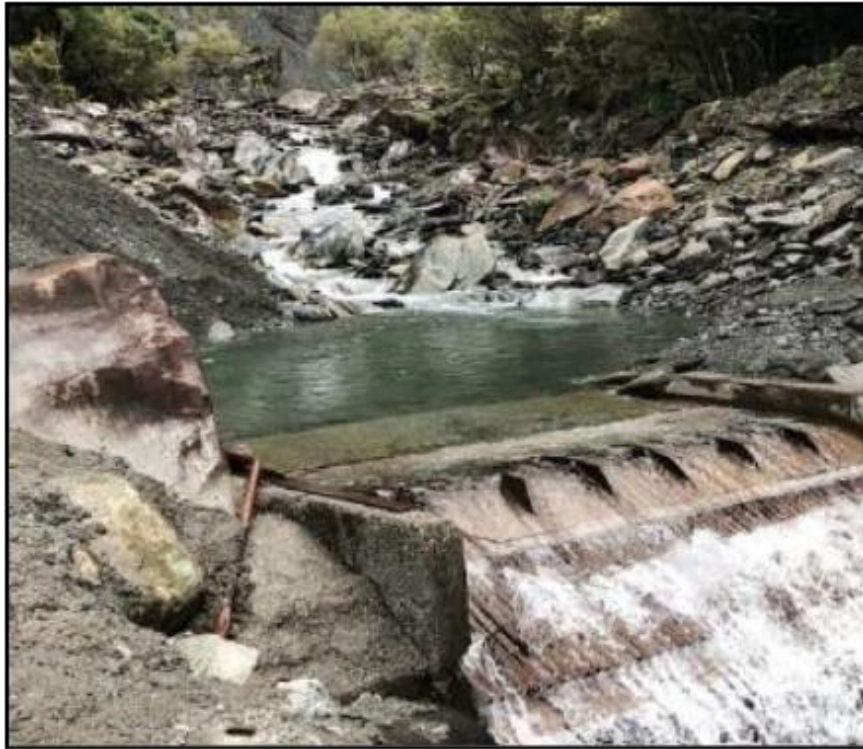
Figure 3-19: Picture of a Tyrolean Weir in an alpine environment (Source: Stantec, 2026).
