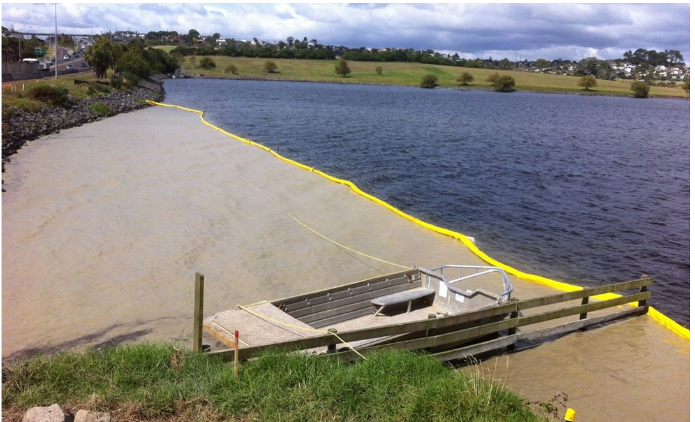
Figure 17 Example of floating sediment curtain ( https://cirtexcivil.co.nz/products/silt-control/envirosieve-turbidity-curtain/ )
