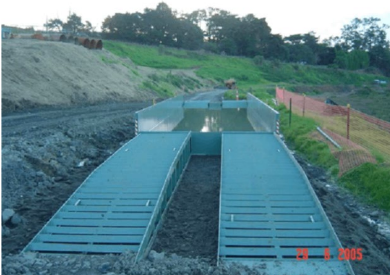
Figure 16 Example of shaker ramp provided by ECAN in the Erosion and Sediment Control Toolbox.
