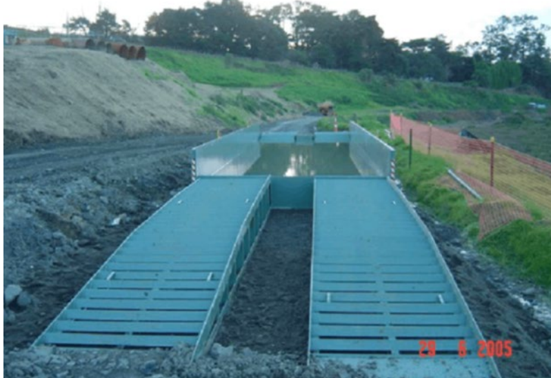
Figure 16 Example of shaker ramp provided by ECAN in the Erosion and Sediment Control Toolbox.
