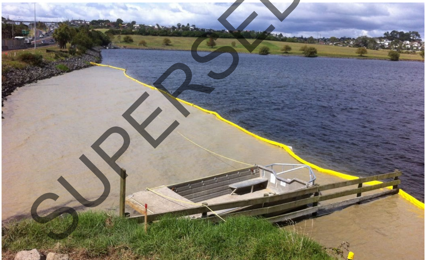
Figure 17 Example of floating sediment curtain ( https://cirtexcivil.co.nz/products/silt-control/envirosieve-turbidity-curtain/ )
