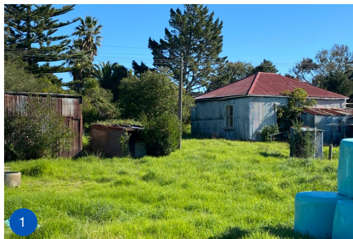
Existing unoccupied dwelling adjacent to small farm sheds
