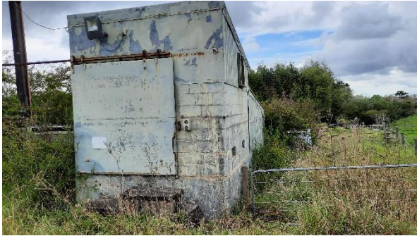
Photograph 3: Livestock farm structure
