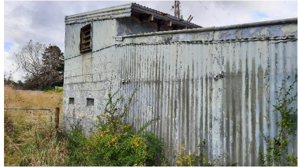
Photograph 4: Southern side of the livestock farm structure
