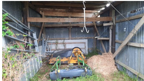
Photograph 12: Inside additional farm building
