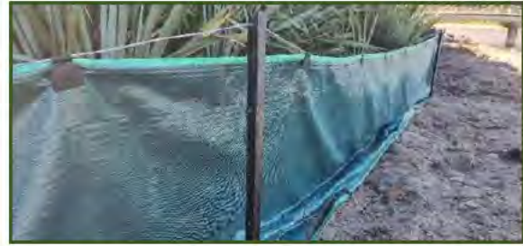
Figure 27: Example of a LEF utilising a sediment control fence (File Photo).
