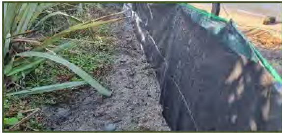
Figure 28: LEF extending >400mm and buried into sand facing the adjacent lizard habitat (File Photo).
