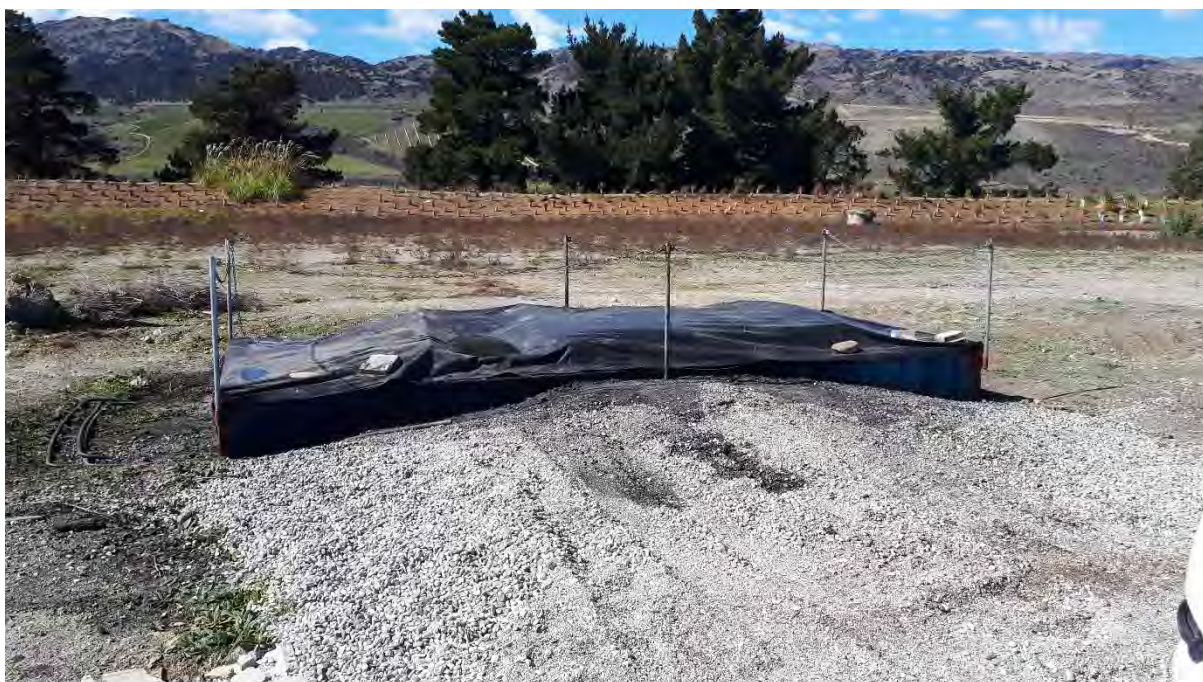
Figure 17: Road cutting waste storage.
