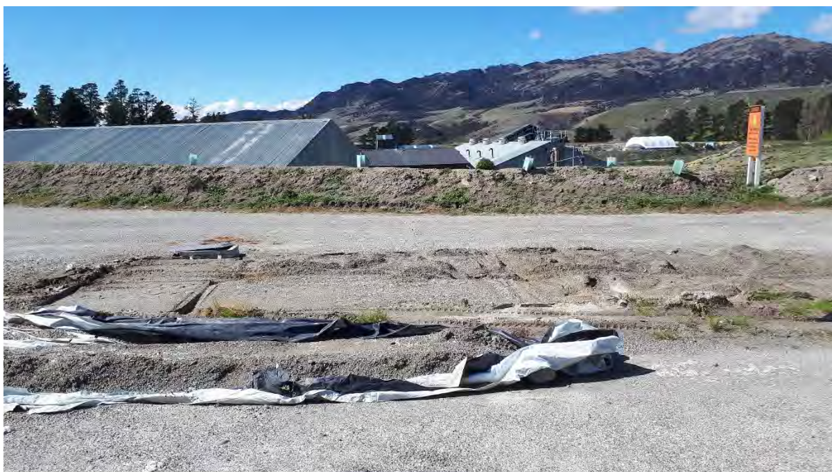
Figure 11: Former diesel tank location.
