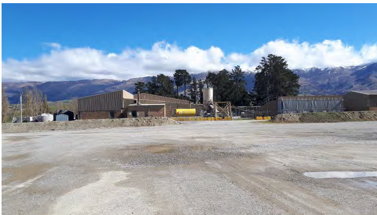
Figure 12: Firth concrete block plant, with concrete silo (white) and diesel tank (yellow) in background.
