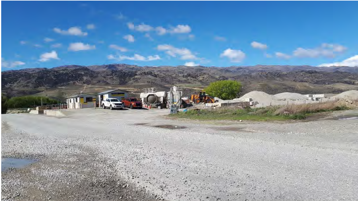
Figure 13: Allied concrete batching plant.
