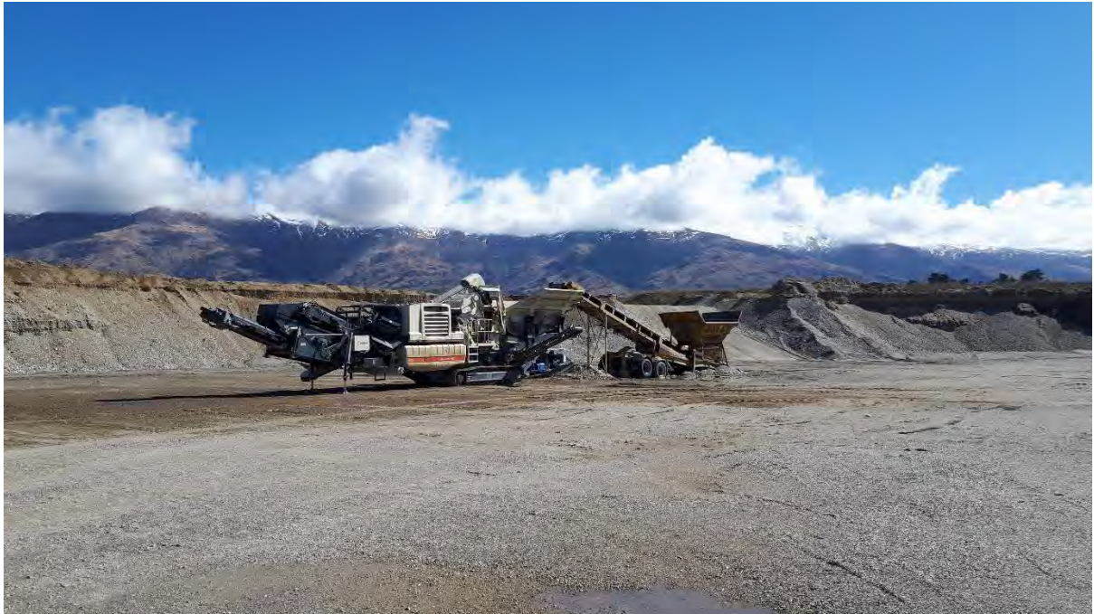
Figure 5: Mobile crusher within Schedule Activity portion of quarry.
