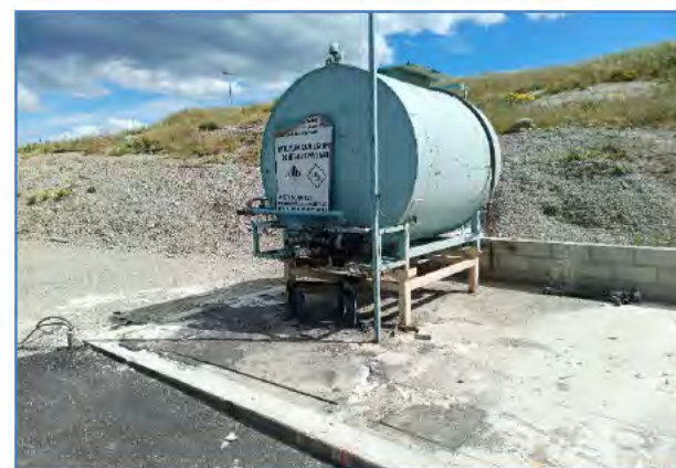
Photo 3: Above-ground bitumen storage tank at the asphalt plant.
