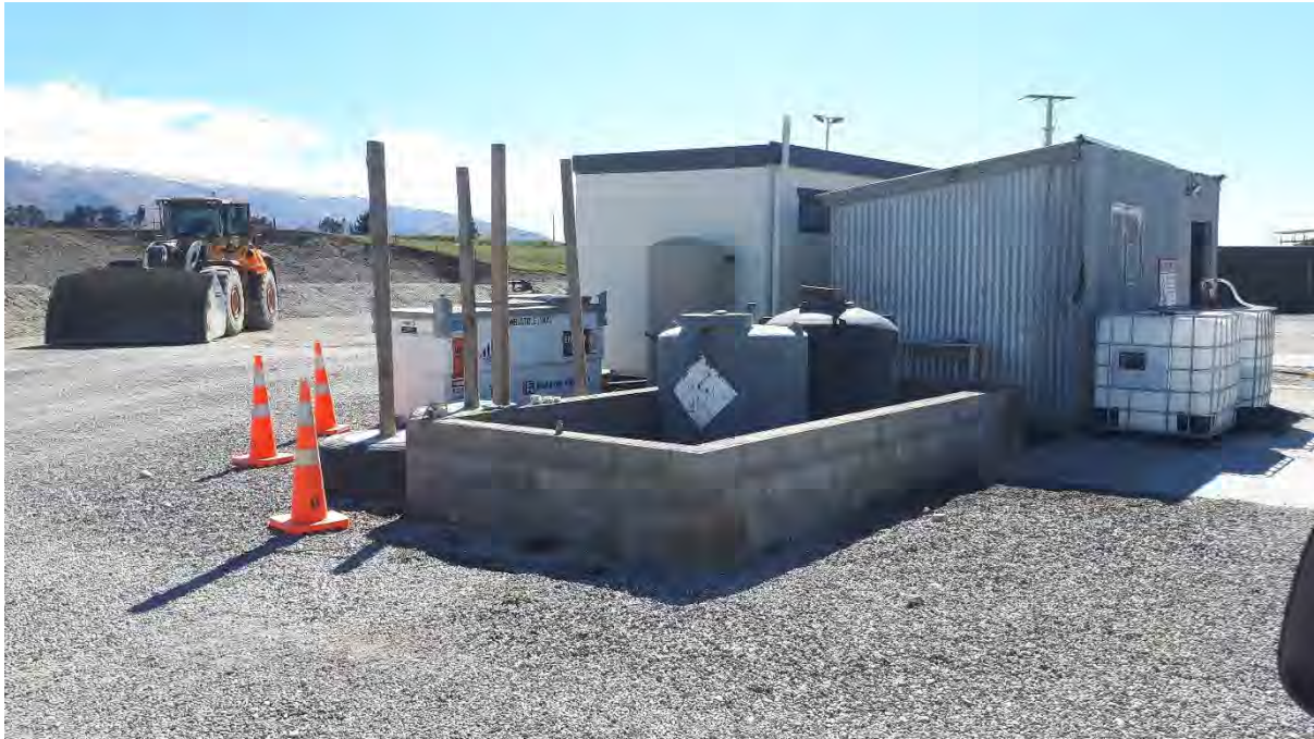
Figure 7: Fuel and waste oil storage within quarry.
