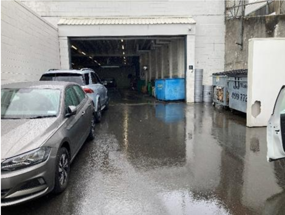
Figure 3 – Gazley Mitsubishi - Former UST location 22-01-2026
