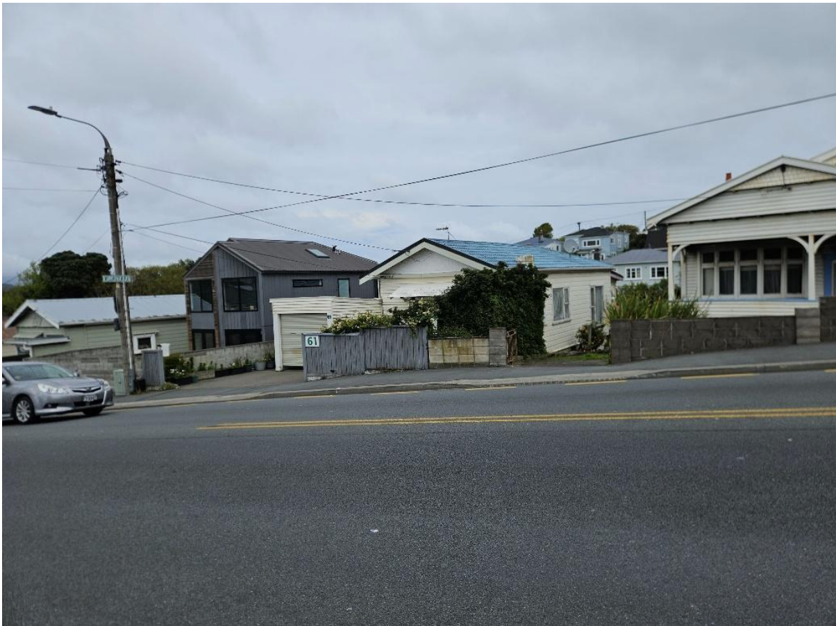
Figure 9 – Residential houses to be demolished on southern side of Wellington Road/SH1 20-10-2025
