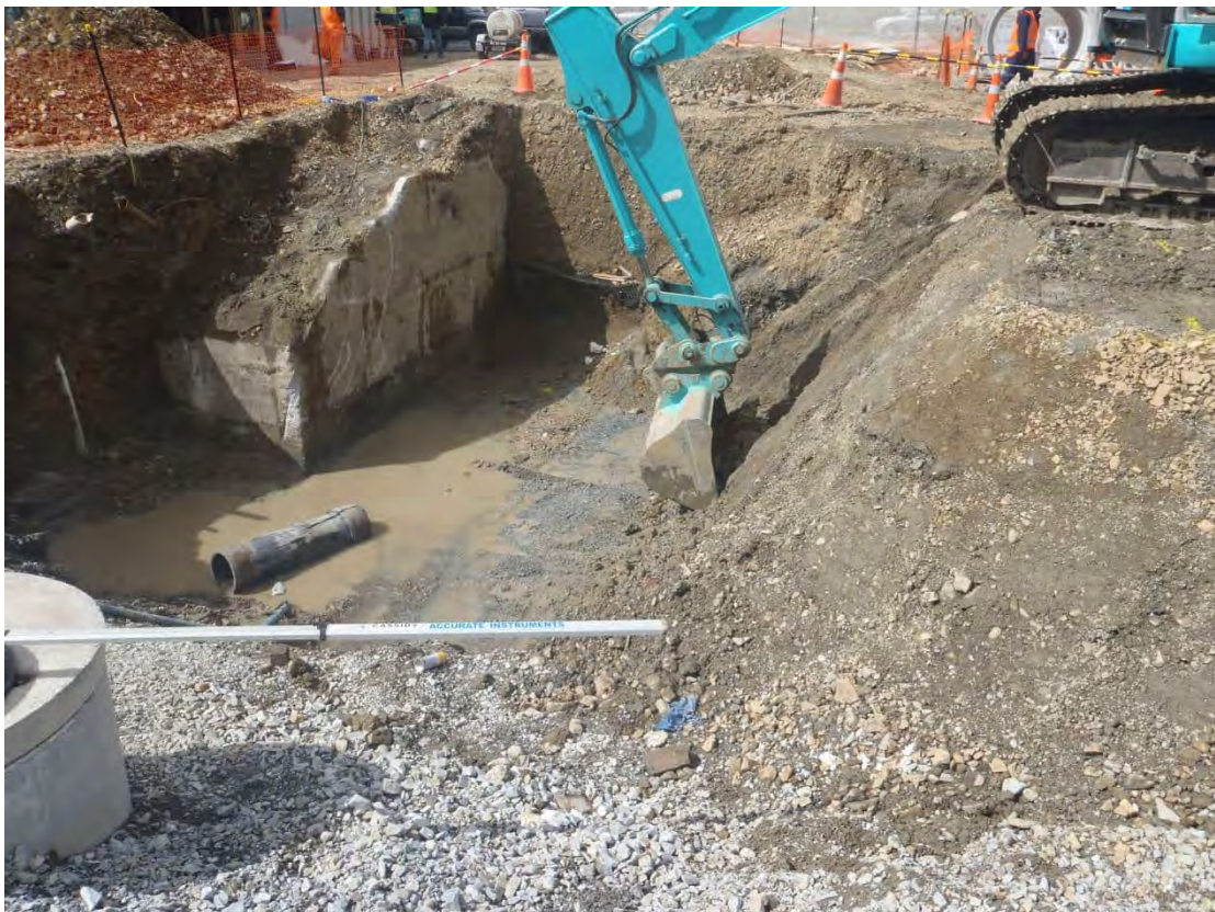
Photograph 12: Looking southeast, canopy excavation (north). Groundwater visible at 3.5 m bgl. Historic UST bund visible in left of shot.
