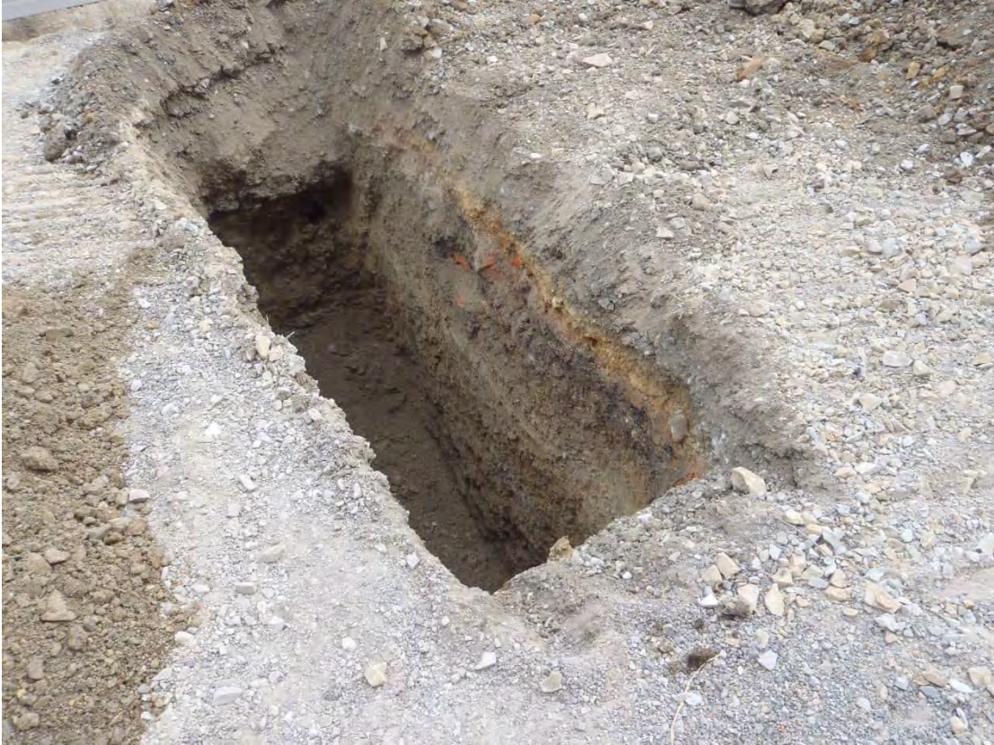
Photograph 3: Test pit 2. Shop excavation. Sandy gravel to 2.5 m bgl.
