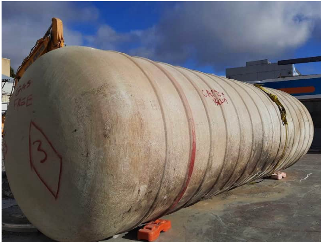
Photograph 2: The photograph shows the 46,000 L diesel underground storage tank. The tank appears to be in good condition.
