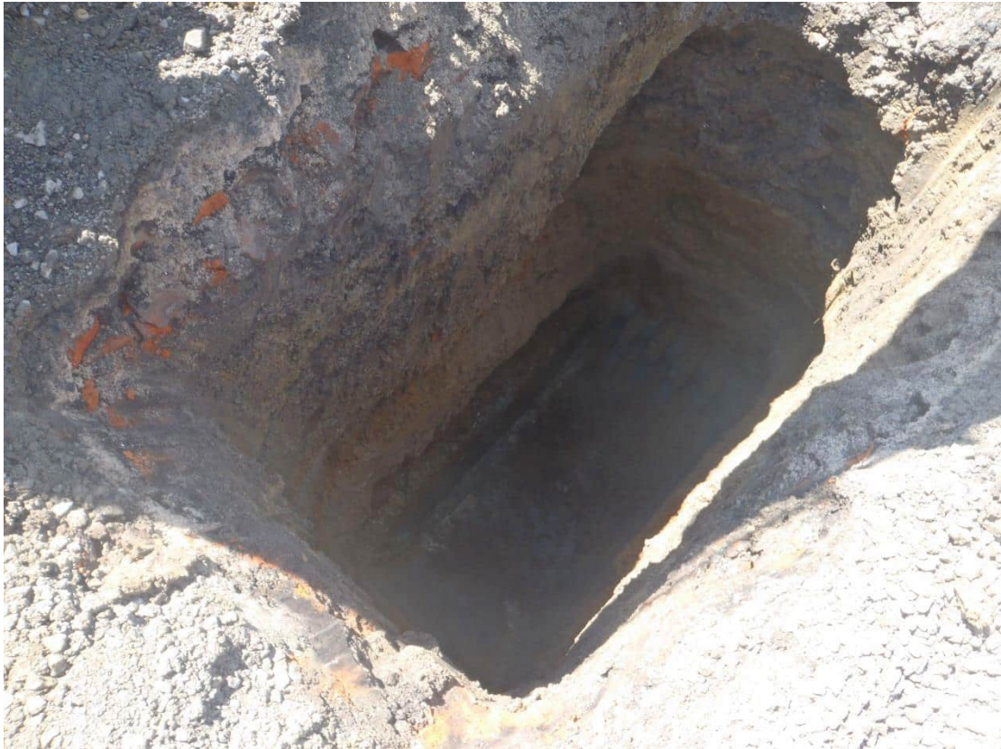
Photograph 13: Test pit 13. Tank pit excavation. Silty clay visible.
