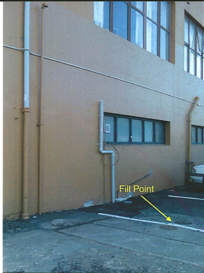
Tank Location looking north-east
