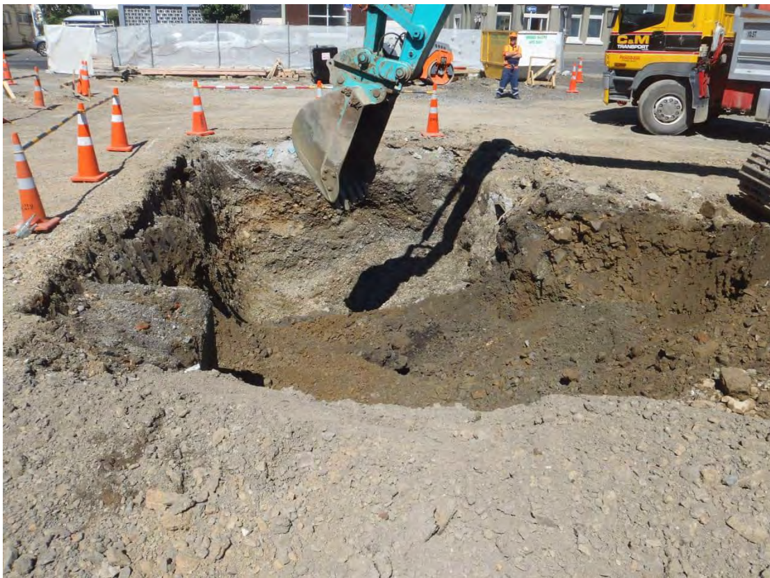
Photograph 6: Looking south, canopy excavation (centre).
