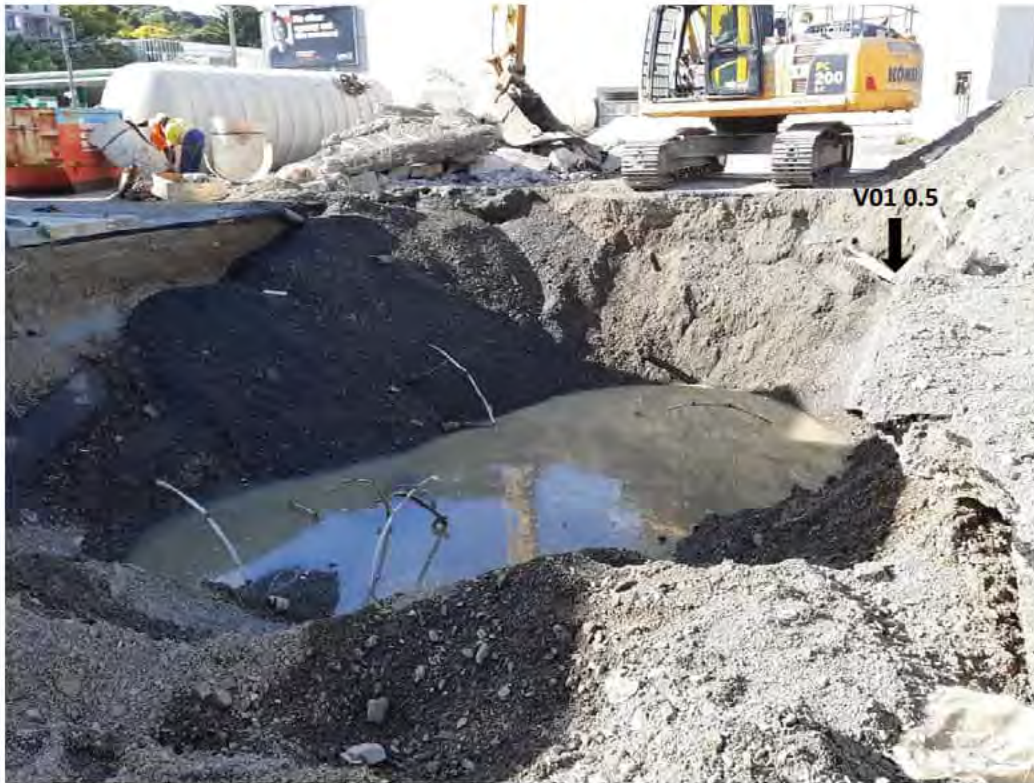
Photograph 3: The photograph shows the tank pit in the north-western corner of the site, from which three underground storage tanks were removed, and the location of the vent risers facing southwest. Groundwater is at about 2.5 m bgl.
