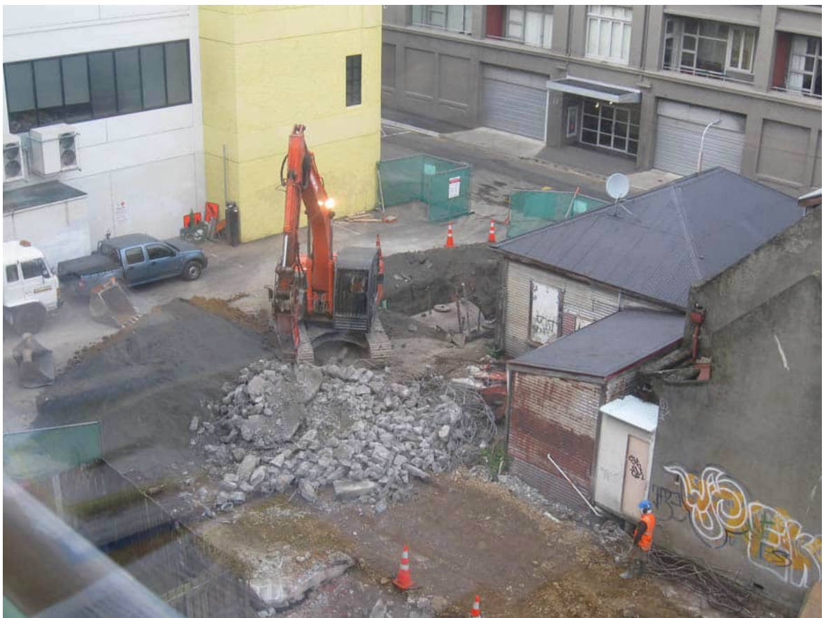
Photograph 2: Location of Tank Pit 1 To the rear of the two bay garage. Back of the historic church on extreme right.
