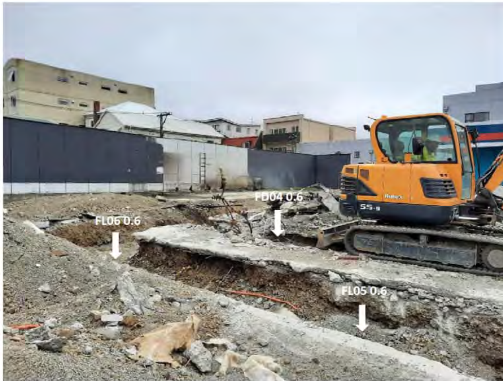
Photograph 5: The photograph shows the former location of the fuel lines and fuel dispensers, facing northwest.
