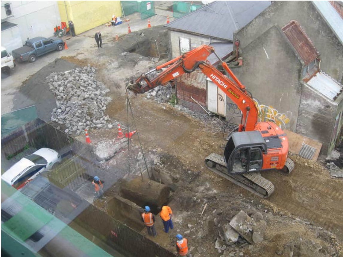
Photograph 5: Location of Tank Pit 3. Removal of one of the 2,000 L USTs from concrete banded pit.
