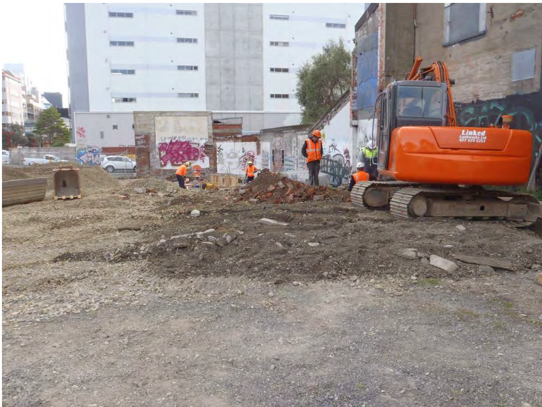
Photograph 2: Looking north, area of shop excavation.
