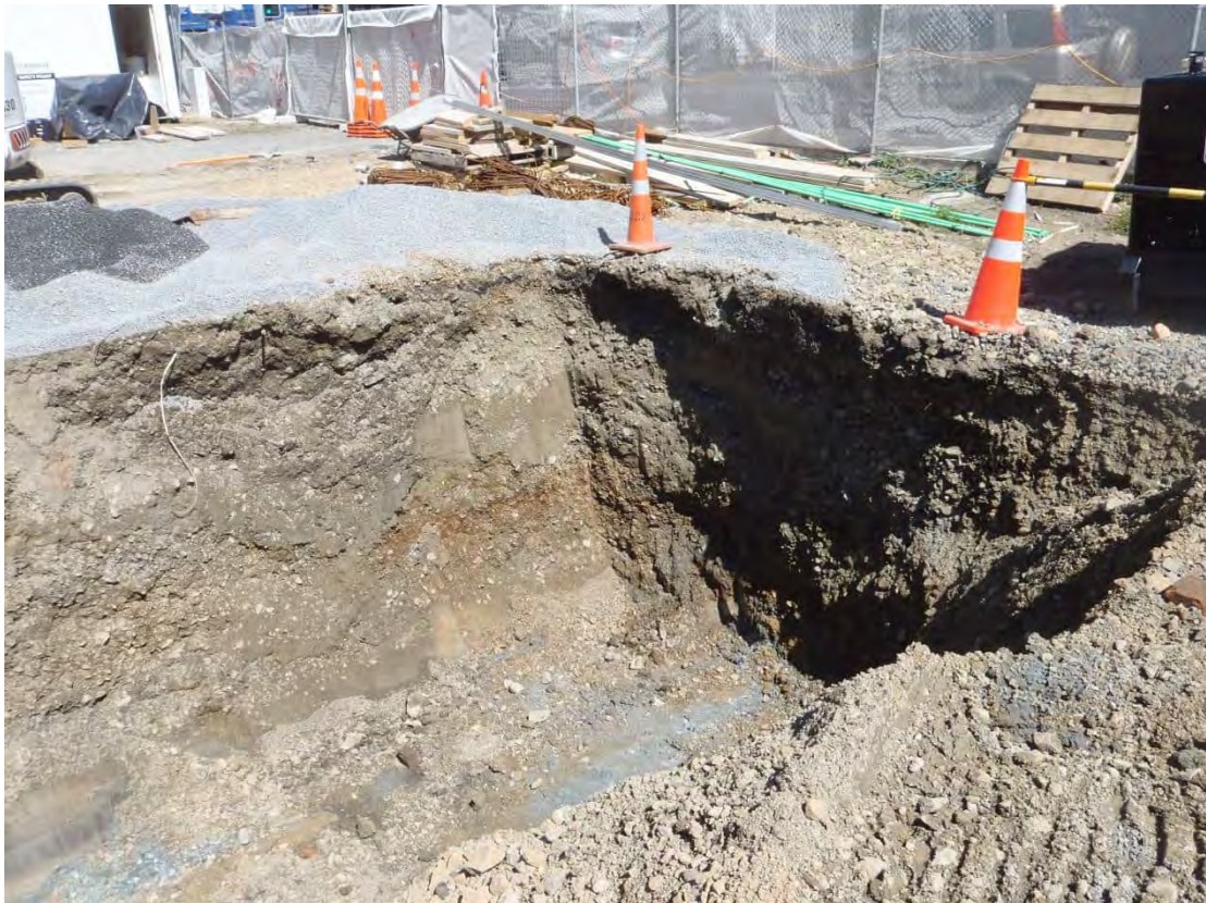
Photograph 10: Looking southeast, canopy excavation (south).
