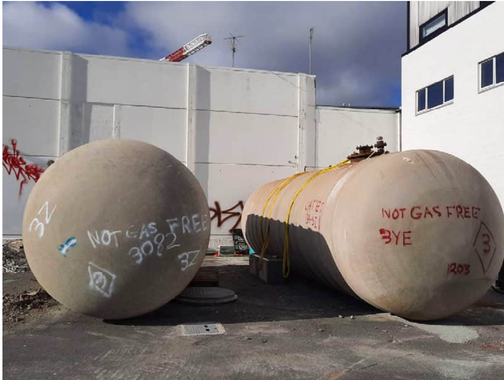
Photograph 1: The photograph shows the two 40,000 L underground storage tanks. The tanks appear to be in good condition.
