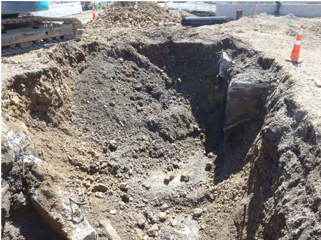
Photograph 8: Looking north, canopy excavation (centre). Historic UST bund visible in right of shot.
