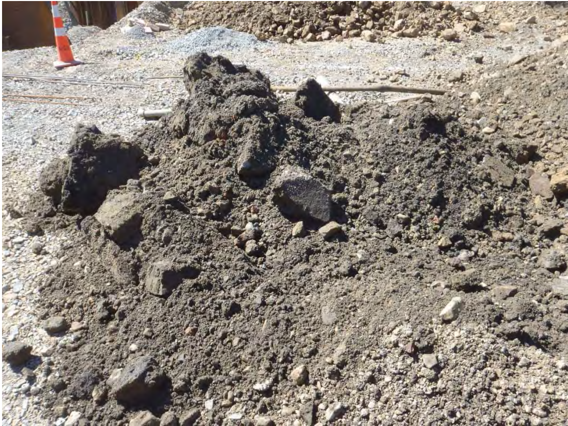
Photograph 7: Material from canopy excavation with dark staining. Excavated from near historic UST bund.
