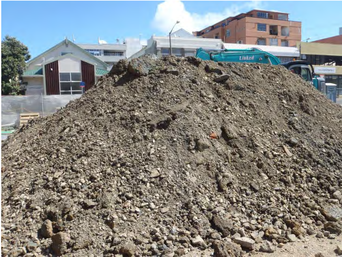
Photograph 11: Material from canopy excavation (south). Predominantly sandy gravel.
