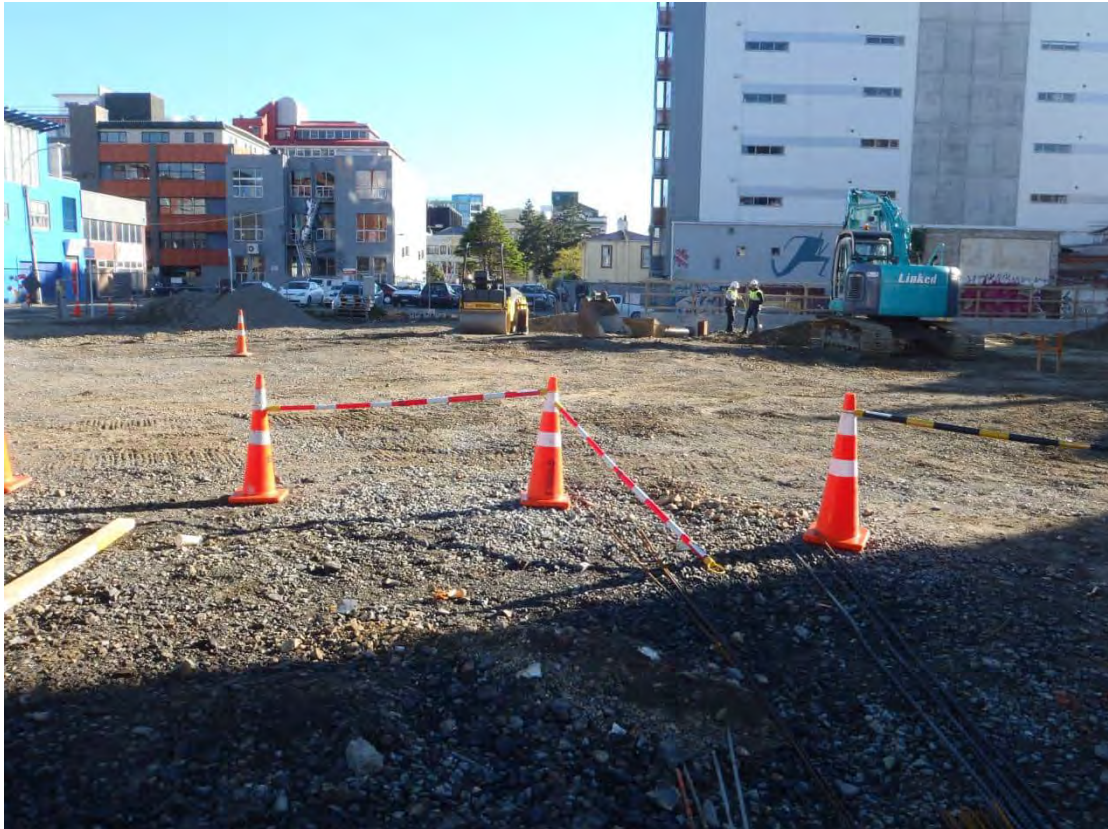
Photograph 5: Looking north, area of canopy excavation.
