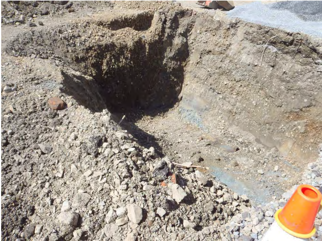
Photograph 9: Looking northeast, canopy excavation (south). Silty clay visible at base of excavation (3.4m).
