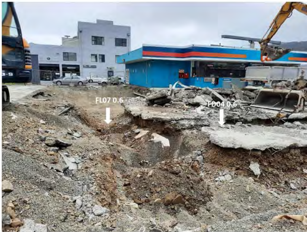
Photograph 6: The photograph shows the former location of the fuel lines and fuel dispensers, facing north.
