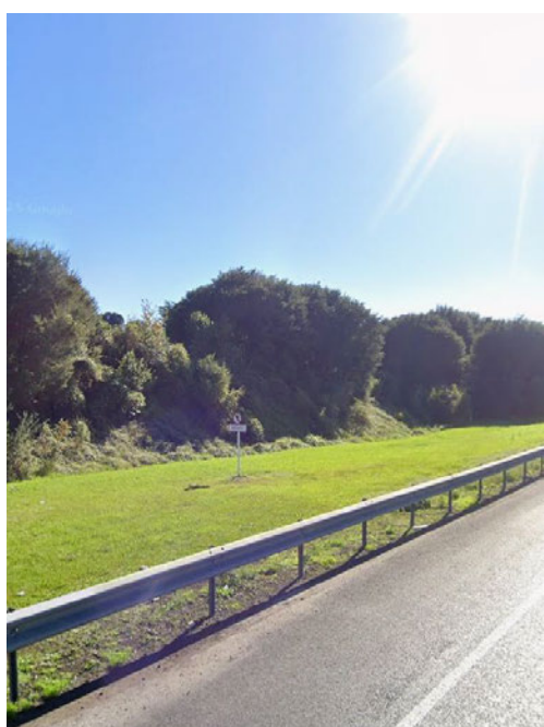
Image 24: Community 9.3 – SH29 roadside screening (west of road)
