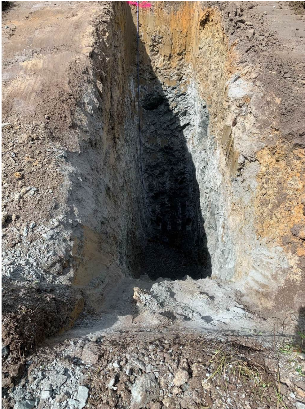
TP22-24 – TEST PIT EXCAVATION
