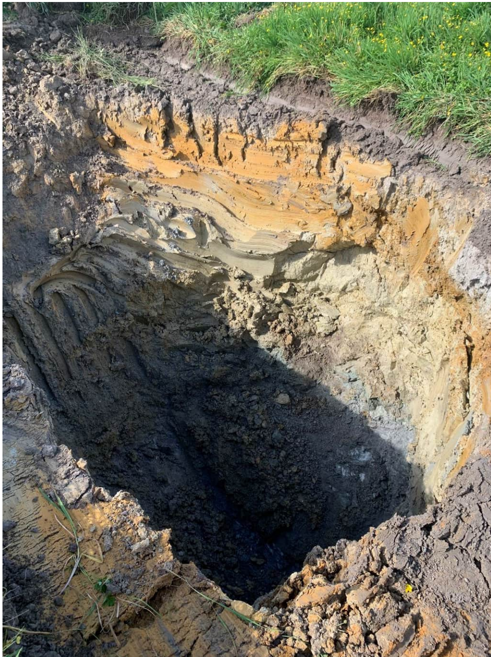
TP23-24 – TEST PIT EXCAVATION
