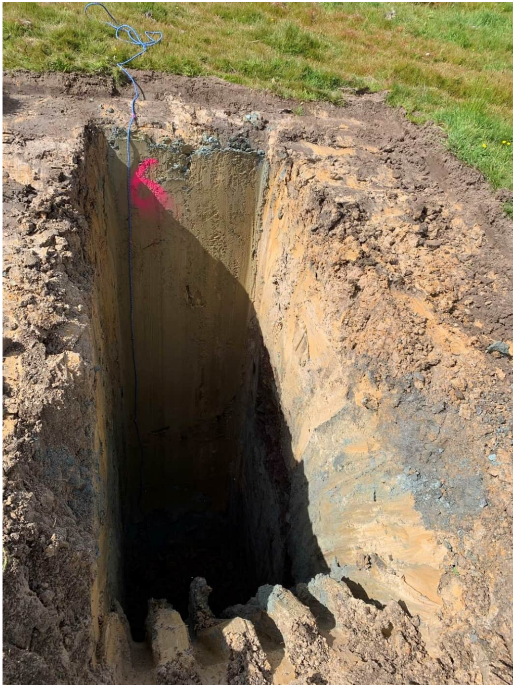
TP06-24 – TEST PIT EXCAVATION
