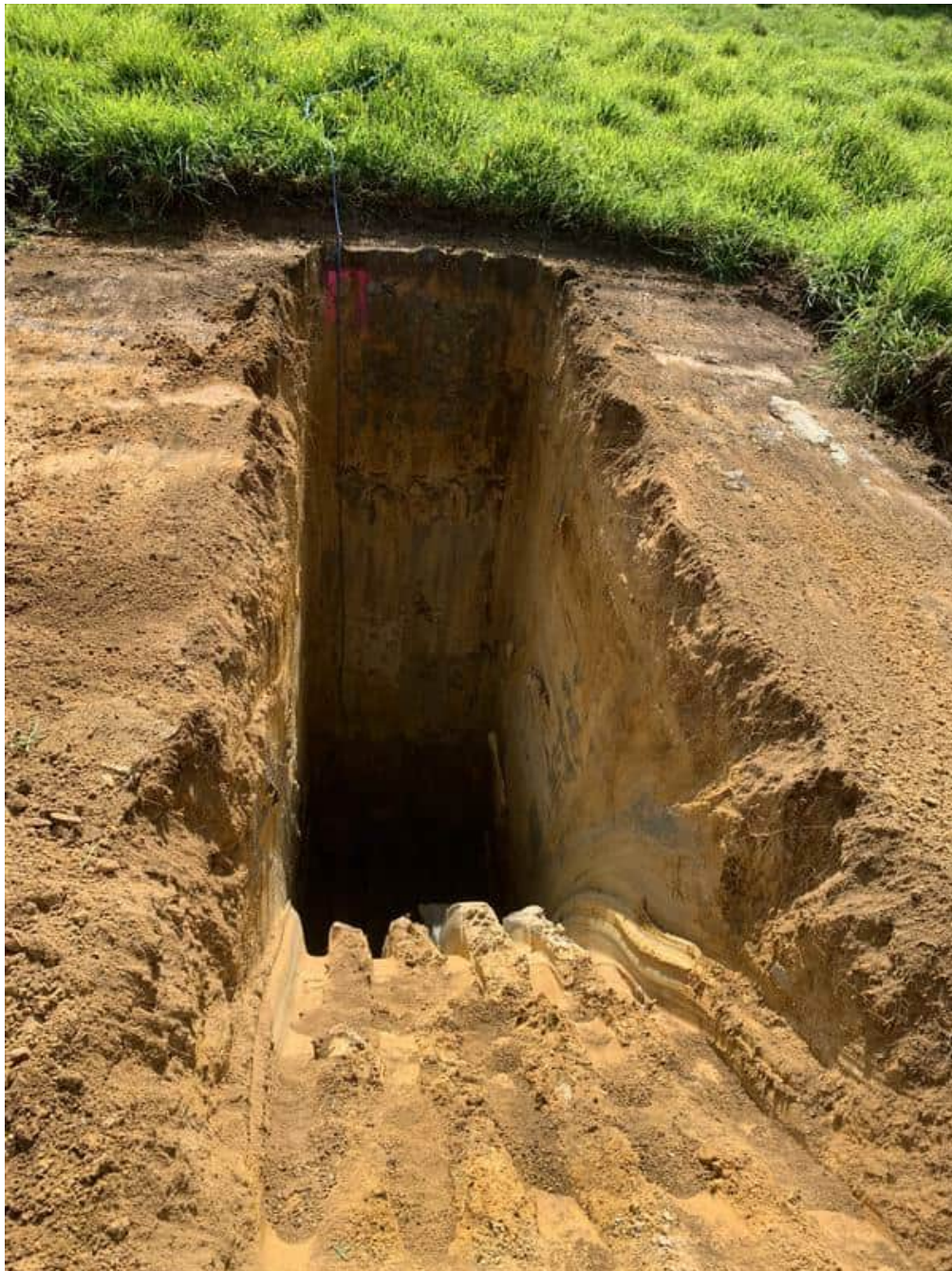
TP17-24 – TEST PIT EXCAVATION
