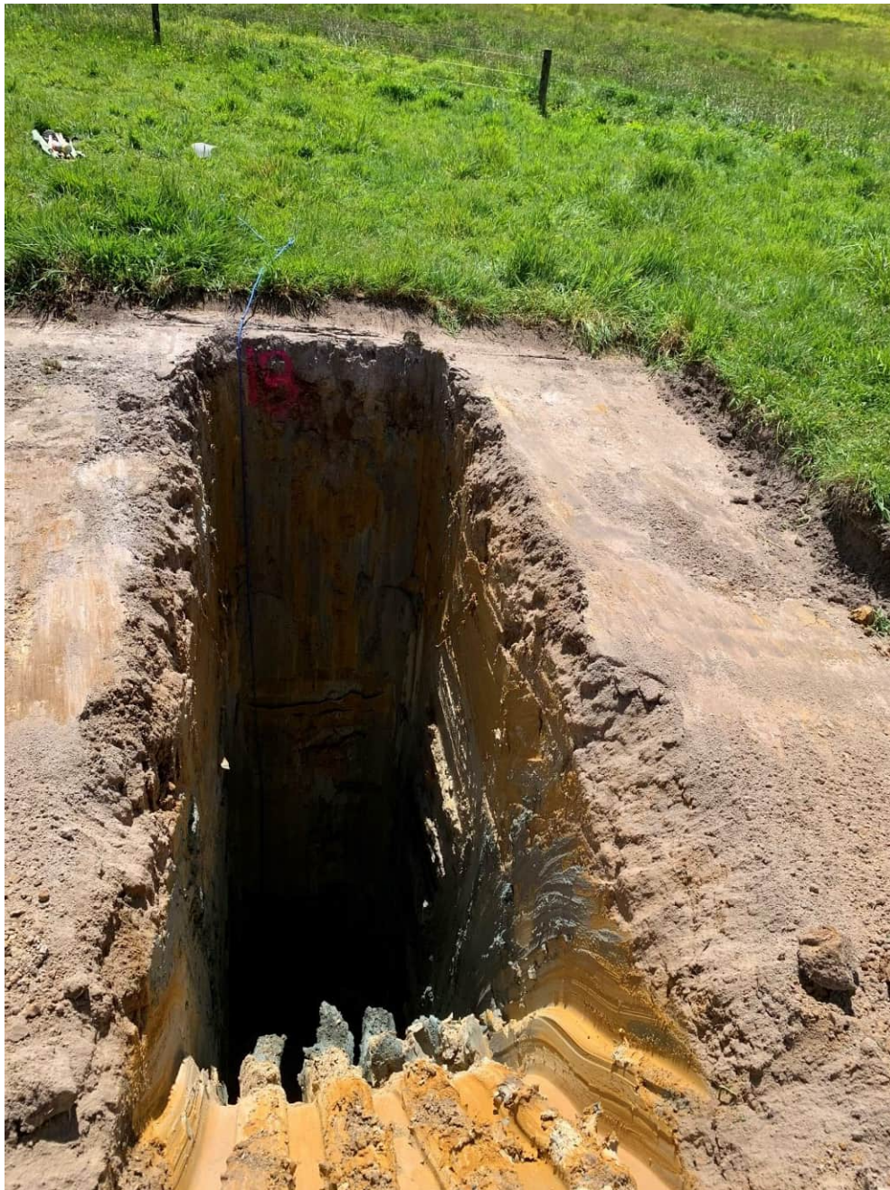
TP18-24 – TEST PIT EXCAVATION
