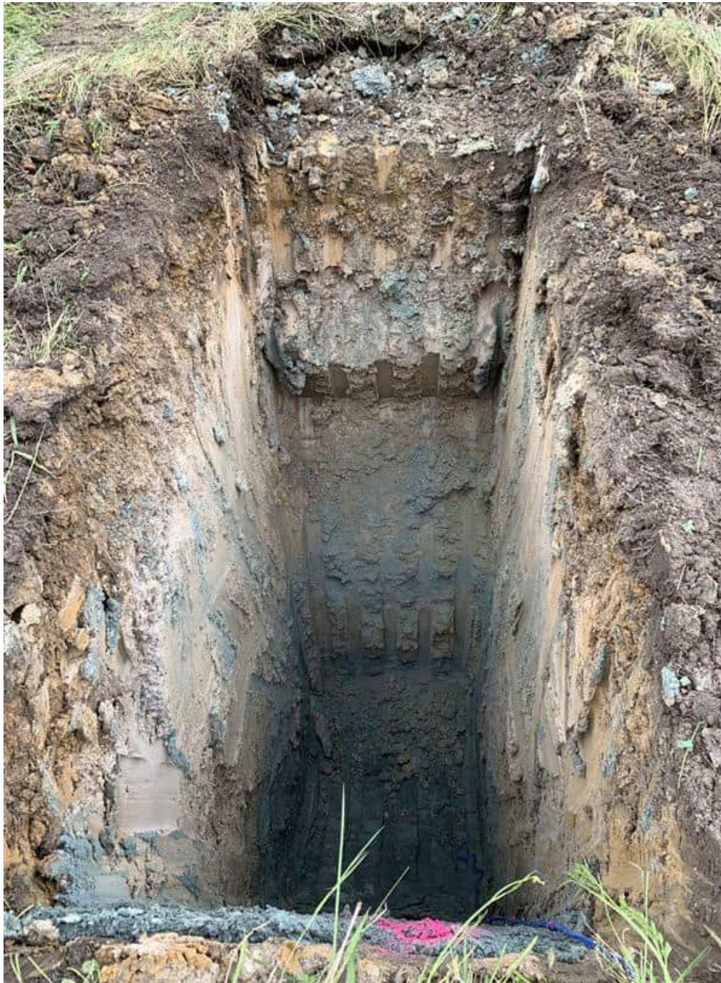
TP01-24 – TEST PIT EXCAVATION
