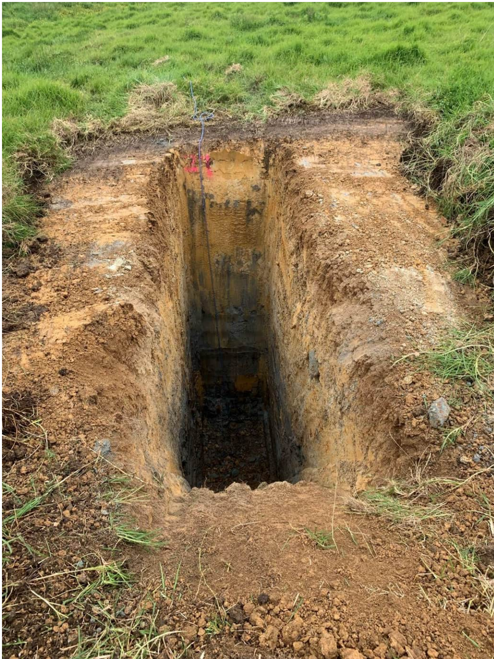
TP27-24 – TEST PIT EXCAVATION
