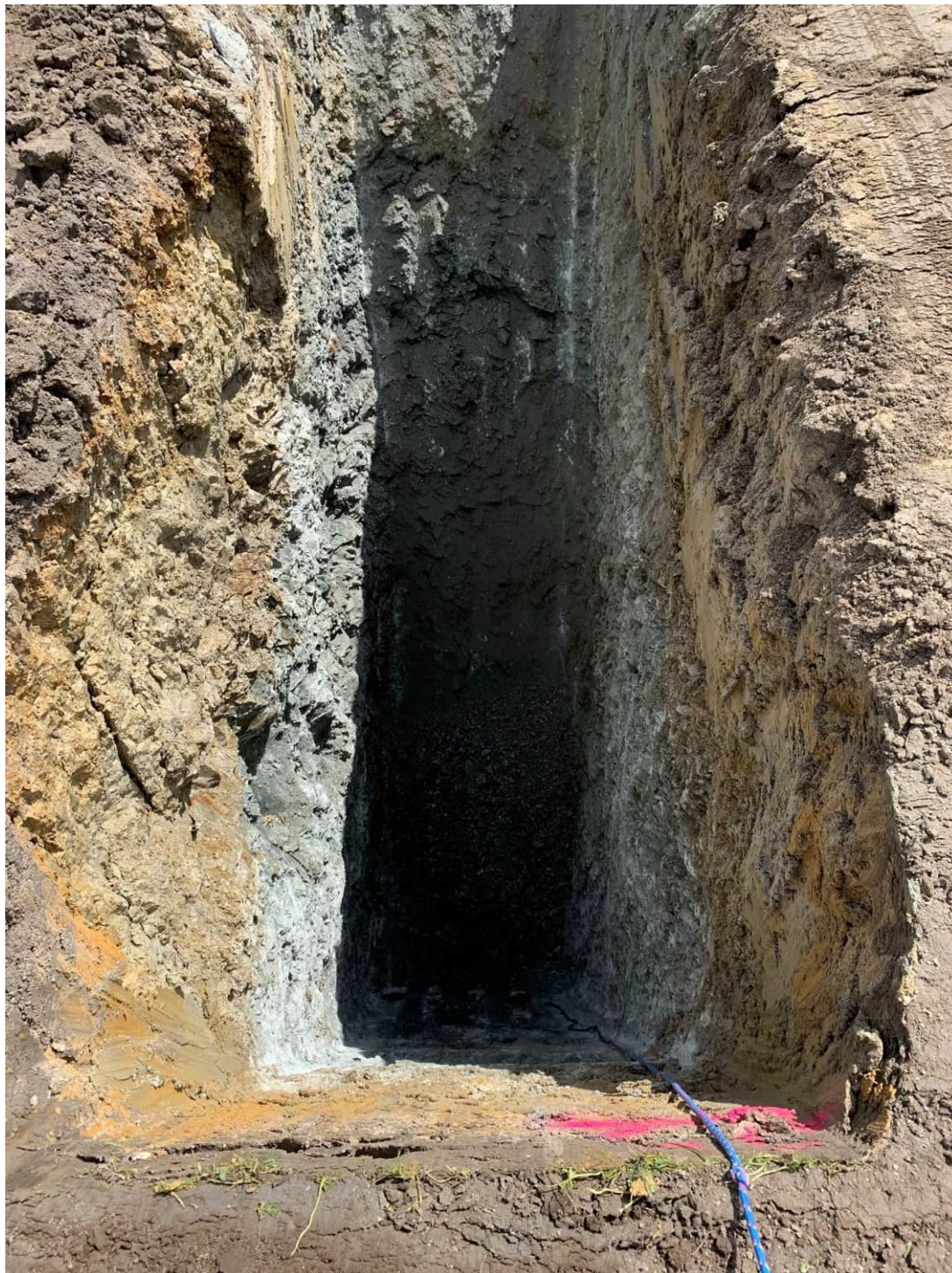
TP22-24 – TEST PIT EXCAVATION
