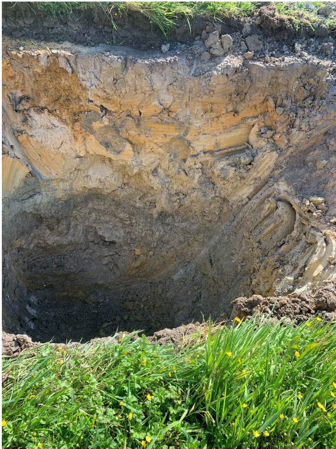
TP23-24 – TEST PIT EXCAVATION
