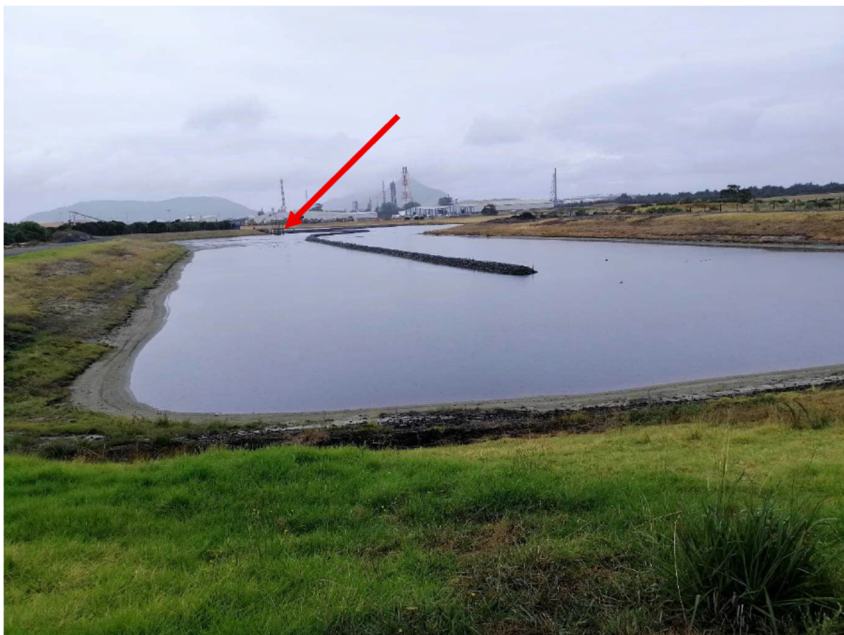
Figure 1: Southern portion of Northport pond with pump station (arrowed) – looking E
