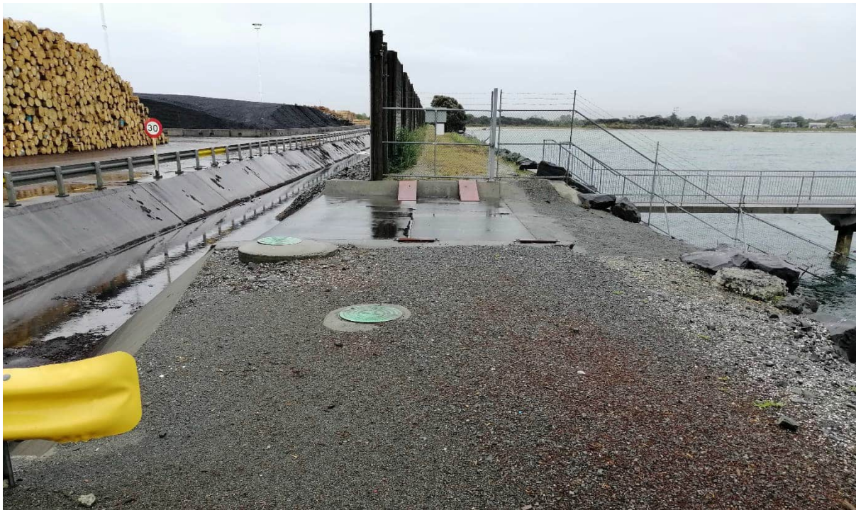
Figure K: Existing Spillway 1 current configuration, ie prior to the new Northport consent modifications being enabled
