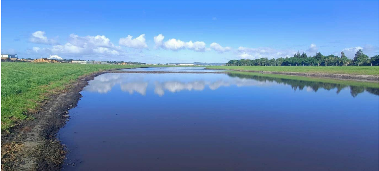
Figure F: Northport treatment pond with forebay baffles – view SSW approx.
