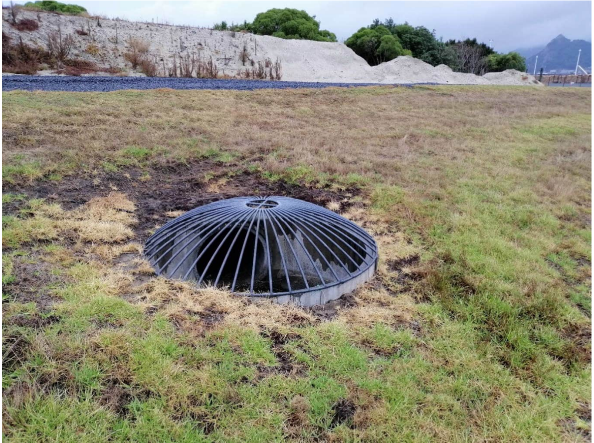
Figure D: Northport pond overflow inlet
