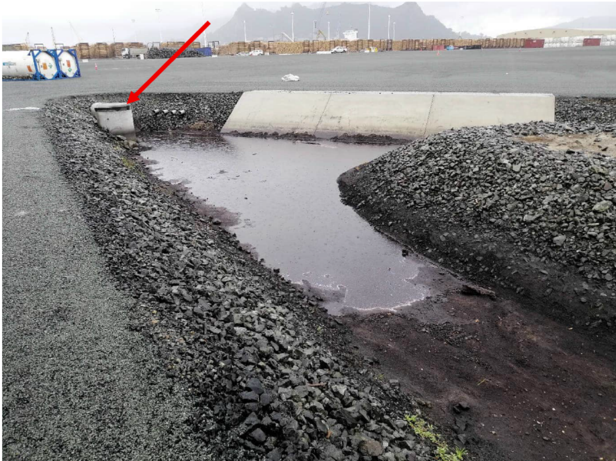
Figure L: Junction of the eastern and western Northport canals with 1200dia culvert outlet constraint (arrowed)
