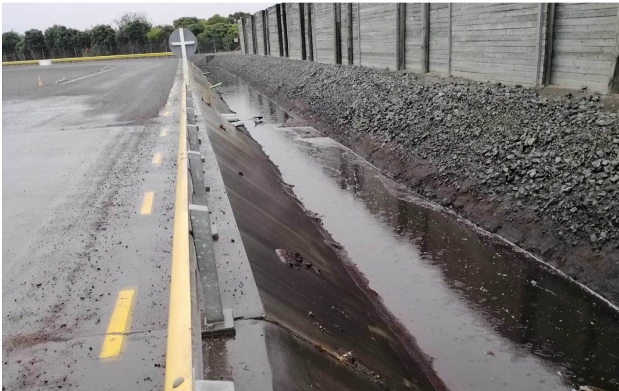
Figure J: Existing Canal 1 at the western limit of the Northport apron – sound attenuation wall to the RHS
