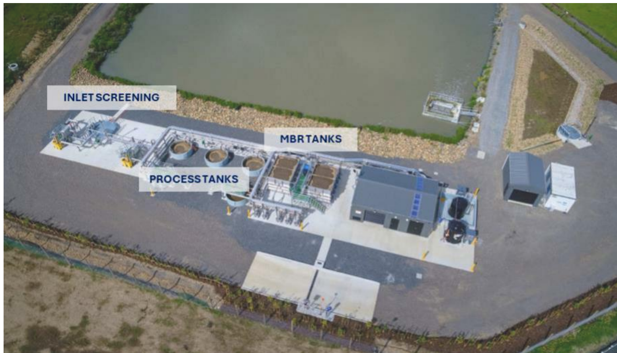
Figure 8: MBR treatment plant designed and built by Apex for Watercare
