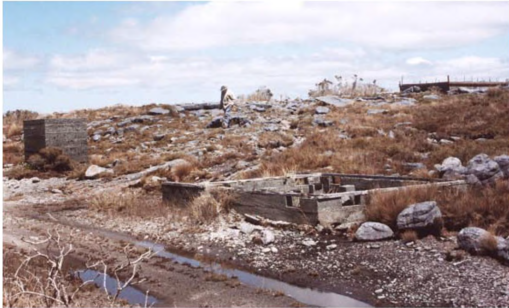
Plate 38: The concrete shell of the Sullivan detonator magazine (36) and the foundation of the original explosives magazine (35). The concrete water tank (34) is on the sky line.
