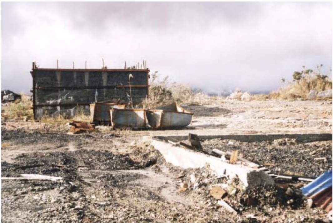
Plate 27: Intact end and side kerbing at Sullivan mine entrance (23), showing recent backfill. The place where the other side kerb was broken off is in the right foreground. In the background, behind the bodies of some old mine boxes or tubs is the concrete water tank (34).
