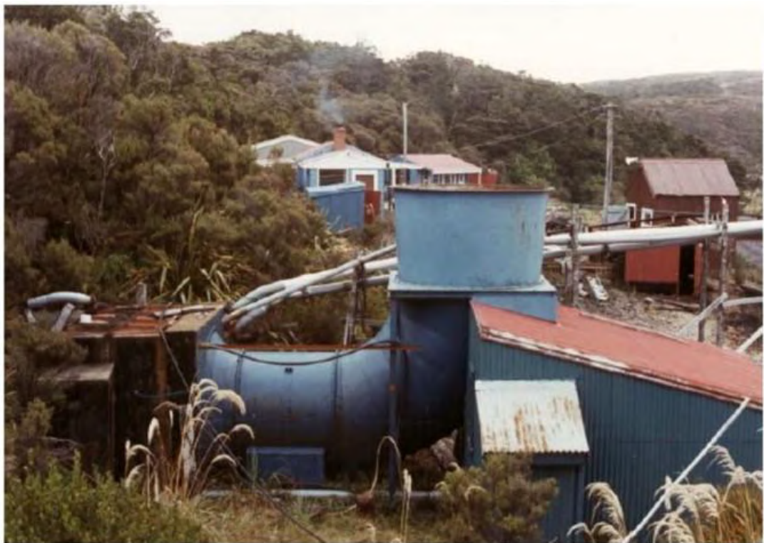
Figure 15. Steps fanhouse during the 1980s with hydro pipes running from the fan drift. In the centre background are the office and workshop, with the store on the stables' foundation beyond and the winch shed at right. In the foreground is the small lean-to pumphouse with a pipe from the dam out of picture at left. (Solid Energy, Westport, photo B2003. in Watson and Wright May 2004:62)
