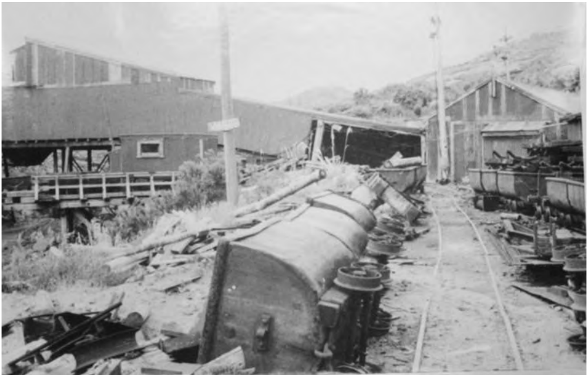
Figure 13. Southward view at Whareatea showing the conveyor gantry with the higher roof built to accommodate the modifications of 1968 at left and the truck loading hoppers just visible below it. Left of the post carrying the 'Whareatea' sign is a footbridge spanning the creek. The mine entrance building is in the right background. (Friends of the Hill in Watson and Wright May 2004:65)
