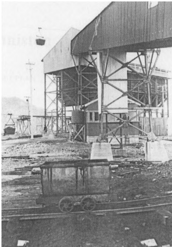
Plate 34 (left): Sullivan conveyor gantry (25) and bins (26) during the pre-1968 period. At left a loaded bucket leaves the bins for the brakehead while an 'empty' passes over the roof of the bins, bound for the Whareatea. The space between the gantry foundations (25b) and tensioner (25c) has yet to be filled by the landing platform (30). The winch house (29) is partly visible.
