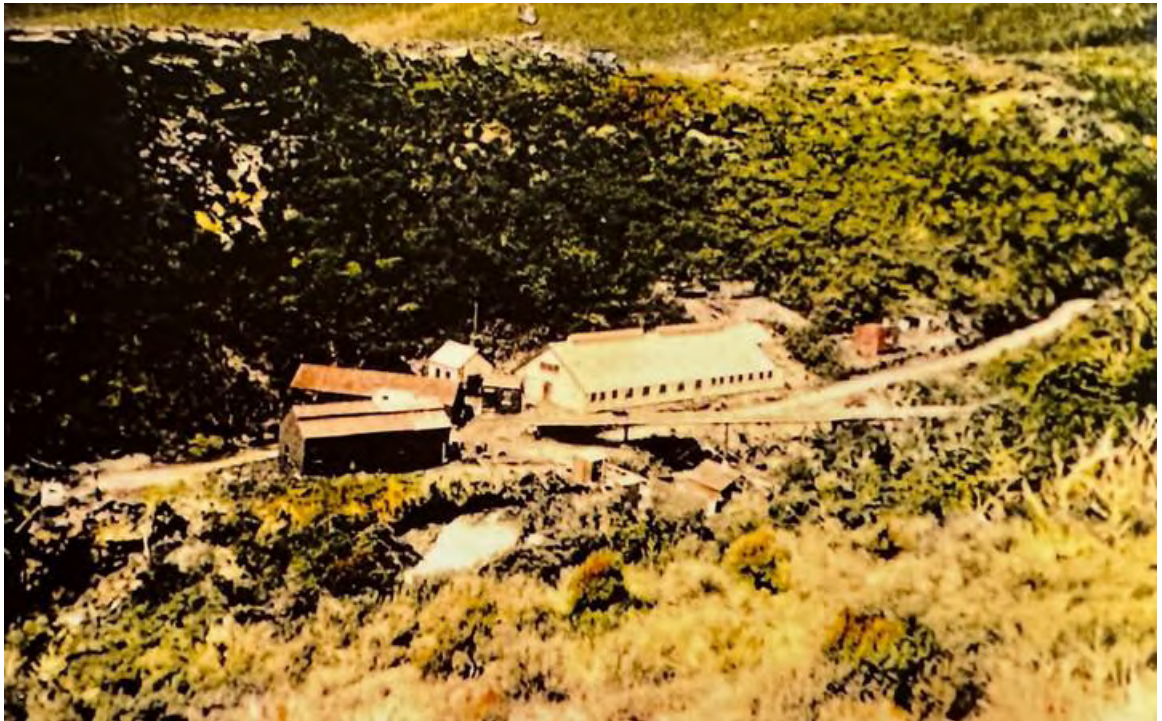
Figure 26. Looking down on Iron Bridge Mine infrastructure. On the left is a toilet, left is the blacksmith's shop and stables, an iron-roofed mine entrance in the centre and a white bathhouse in the right. The bridge on the right goes to Burnett's Face (source: Bill Andrew Collection, Friends of the Hill)
