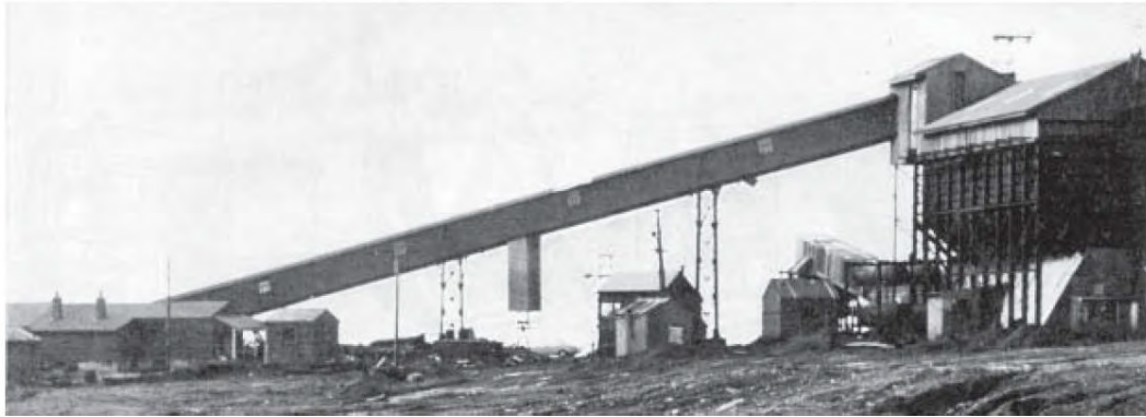
Plate 33: The Sullivan mine from the south in 1977 with the mine conveyor gantry (25) going up to the bins (26) at right and the smaller gantry (27) connecting with the truck loading bin (28) beyond. At centre is the conveyor belt tensioner (25c) with gantry supports (25b and 25c) on either side. The winch shed (29) is right of the tensioner with the electrical substation (31) nearer the camera and the compressor shed/garage (33) farther right again, mostly obscuring the truck bin. At left are the mine offices which have disappeared entirely. (Peter Robertson photo from 'New Zealand Coal' Vol. 21: No. 4: Spring 1977.
