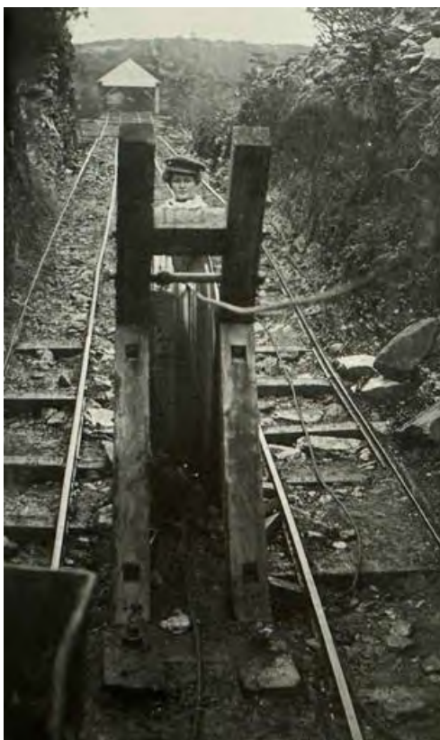
Figure 32. Kiwi Mine jig for the rope road (source: Series PA1-o-990, #20, Alexander Turnbull Library, Wellington)
