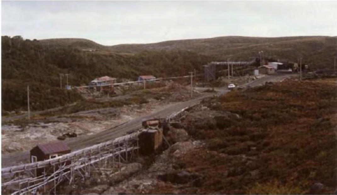
Figure 14. A northward view of the Whareatea fines filtration tank with flumes from the Escarpment (left) and Whareatea pads visible, along with hydro pipes and the pump shed at left. The mine offices and workshop and the storeroom on the stables' foundation are farther back, left of centre beyond the hydro pipes from the mine. (Solid Energy, Westport, photo B2002 in Watson and Wright May 2004:71)
