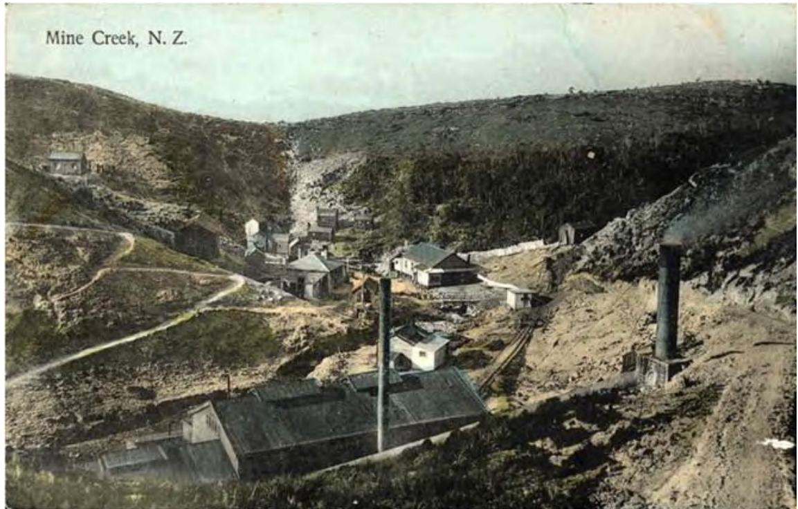
Figure 44. View down into Mine Creek, from the west of the settlement. The boarding house is the main building, as well as other various sheds/huts. A tramway can be seen heading south from the aforementioned large building, and has coal tubs on it. The mine entrance can be seen behind this and there are sheds along the line (source: Granity Museum)
