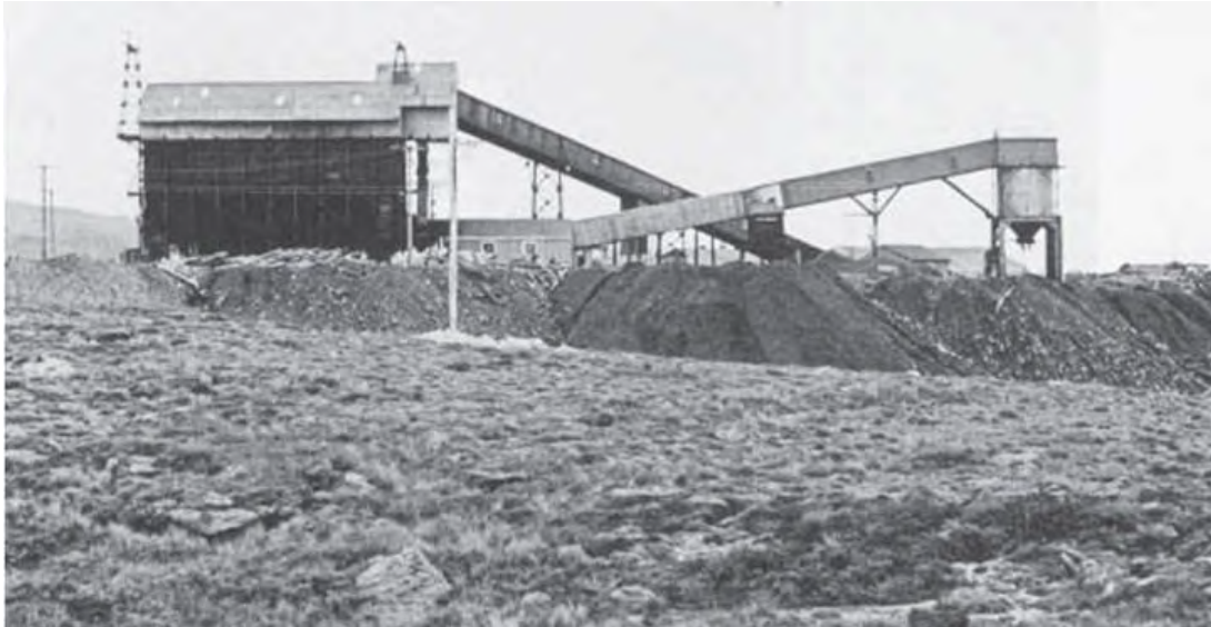
Figure 20. Sullivan bins from the east in 1984 with conveyor gantries to the mine behind and the truck bin at right. To the right of a gantry support, about the centre the mine conveyor tensioner is visible although mostly obscured by the truck bin gantry. Aerial towers still stand on top of the bins. ('New Zealand Coal' Vol. 28: No. 1, Autumn 1984. In Watson and Wright May 2004:74)
