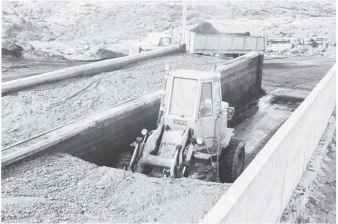
Figure 16. Loading coal from the Whareatea pads. The truck is standing on the lower part of the apron, from where the photo above was taken. (Solid Energy, Westport, photo B2007 in Watson and Wright May 2004:69)
