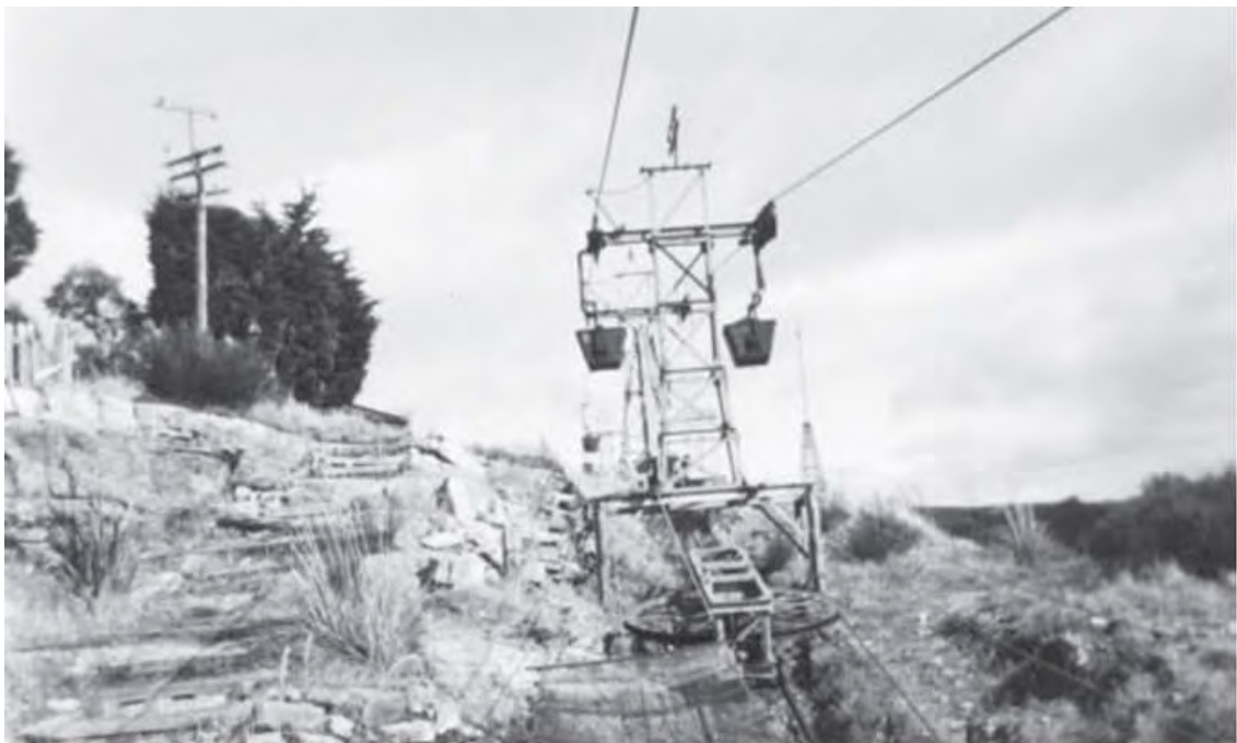
Figure 8. At the brakehead end of the aerial, a complex system kept the cable taut. Many elements of the tensioner (Feature A40) remain, including the large wheel (inset lower right) visible in front of the tower. (Photo courtesy of Brian Kerr. In Watson and Wright May 2004:88)
