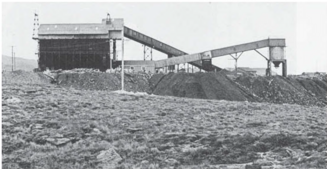
Plate 30: Sullivan bins (26) from the east in 1984 with conveyor gantries (25 and 27) to the mine behind and the truck bin (28) at right. To the right of a gantry support, about the centre the mine conveyor tensioner is visible although mostly obscured by the truck bin gantry. Aerial towers (see Fig. 10) still stand on top of the bins. ('New Zealand Coal' Vol. 28: No. 1, Autumn 1984.)
