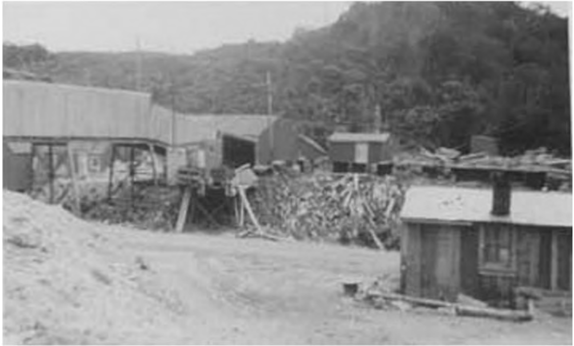
Figure 12. Whareatea c.1960 with the mine conveyor gantry running from the building at the mine entrance in the middle background to the left. The early underviewers' office is to the right of the entrance and the early workshop is at right (Department of Conservation, Westport in Watson and Wright May 2004:65)
