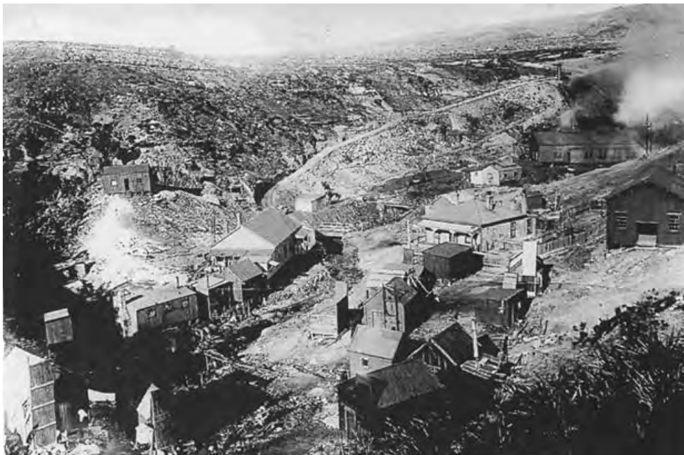
Figure 43. Looking south over the settlement of Mine Creek. The power house and ventilation flue are in the background (right) on the true right of Mine Creek, and a pack track above, which leads down to a bridge over the creek. The boarding house is central with an ornate verandah surrounded by other sheds/huts. There is an industrial looking corrugated iron building on the slope (right) (source: Crawshaw 2000:33).
