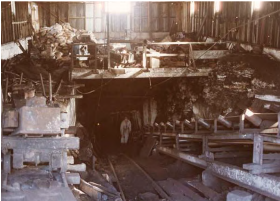
Figure 21. A view down the Sullivan Mine entrance late in the mine's life, with the rails at centre and conveyor at right. Materials and equipment were stored in the large entrance shed (Solid Energy, Westport, photo B2020. In Watson and Wright May 2004:74)
