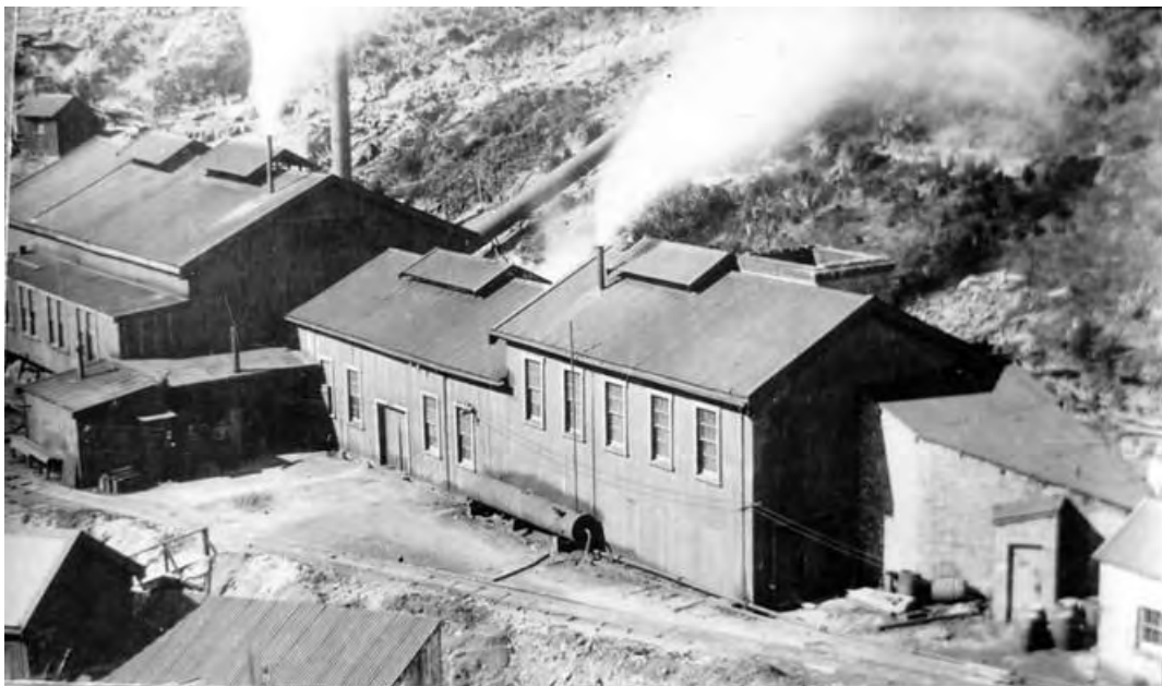
Figure 41. The air compressor and fan drive sheds on the true right of Mine Creek. The square top of the brick ventilation flue is visible behind the fan drive shed, which was home to the Schiele fan. There is a brick or concrete structure to the south of this shed. A metal pipe leading up to the flue is visible on the hillside. There is a rail line between the sheds and Mine Creek. A metal pipe leading up to the flue is visible on the hillside. There is a rail line between the sheds and Mine Creek (source: Coaltown Museum Ref: MN56)
