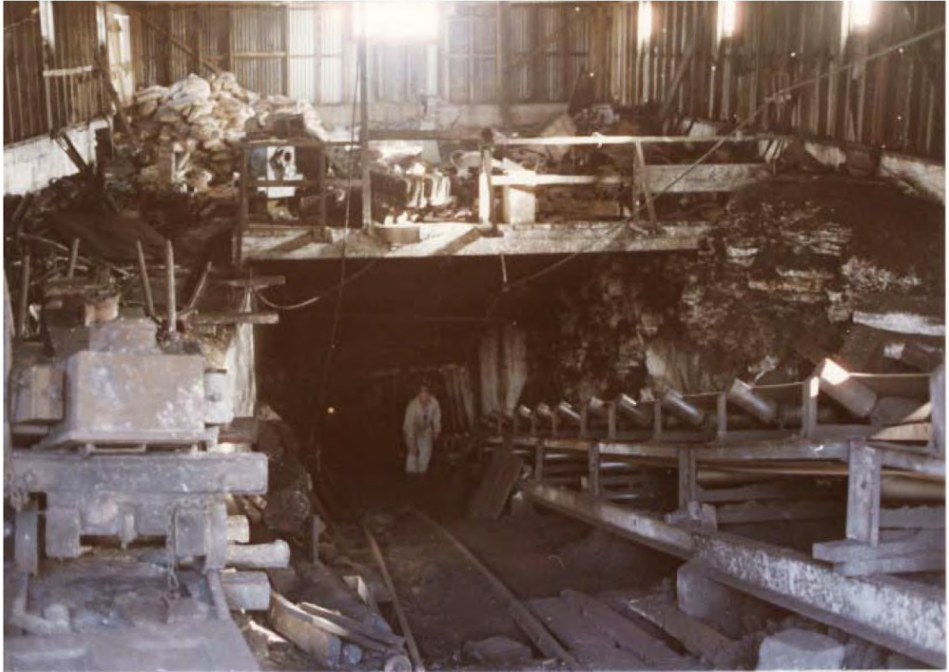
Plate 29: A view down the Sullivan entrance (23) late in the mine's life, with the rails at centre and conveyor at right. Materials and equipment were stored in the large entrance shed. (Solid Energy, Westport, photo B2020.)
