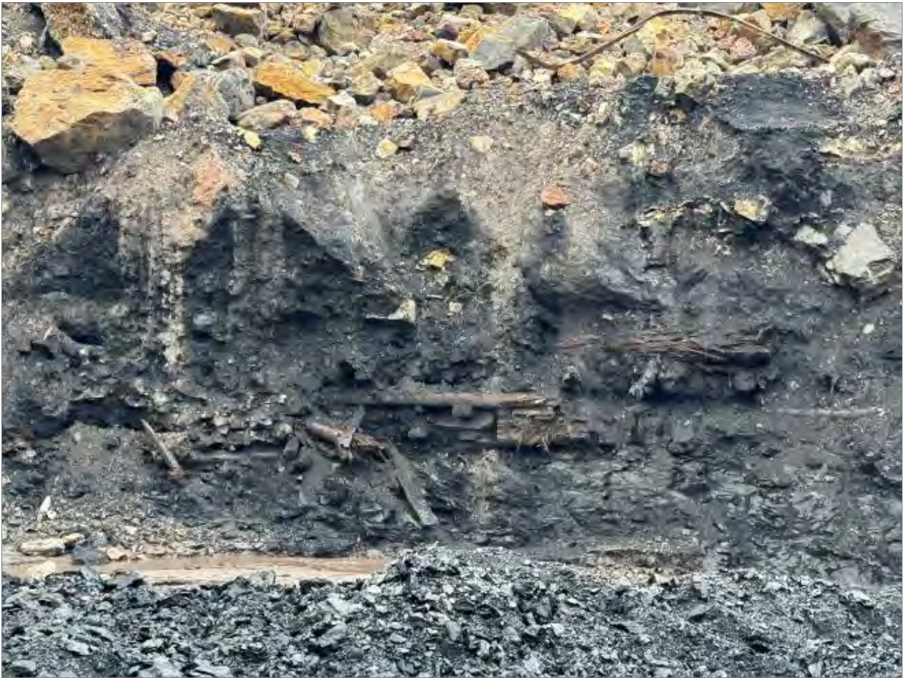
Figure 2.4 Coal Adit collapse at Millerton (source: Bathurst)
