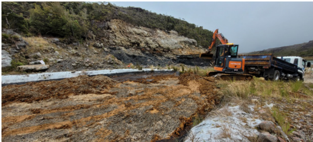
Figure 29: Example of AMD sludge removal from a MSR following reactor dewatering using an excavator.
