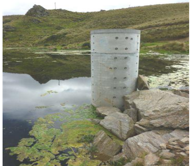
Plate 6. Typical Silt Pond Decant Structure
