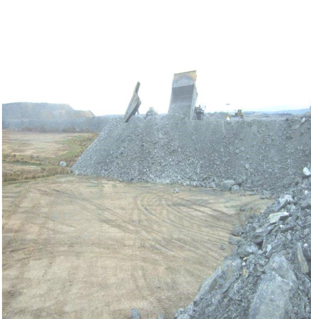
Plate 7. Rock Stack Tip Face (initial lift)
