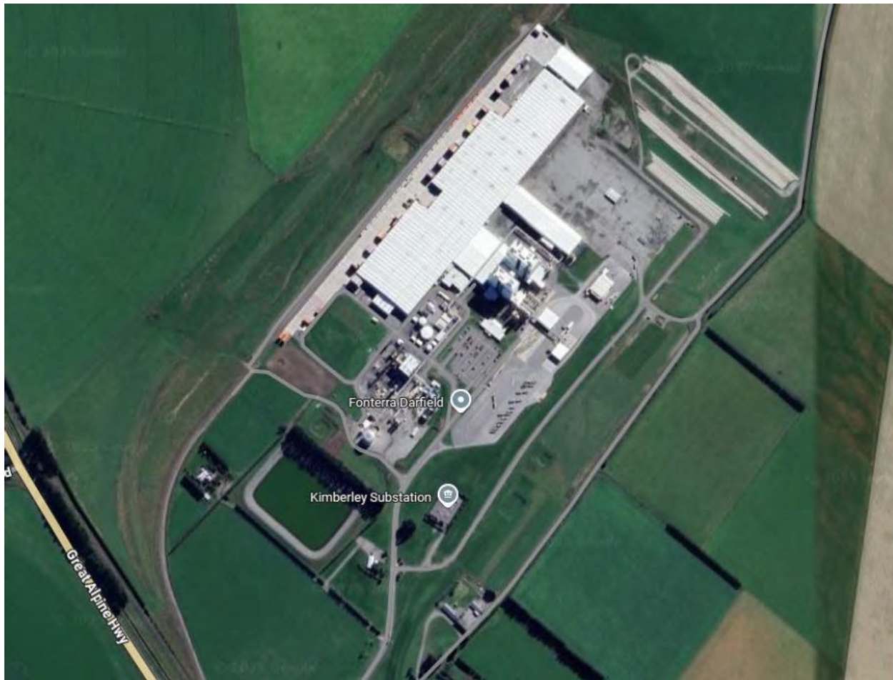
Figure 2.9 – Aerial Image of the Fonterra Darfield Plant
