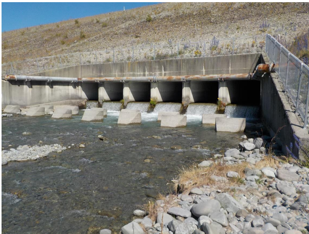
Figure 3: The Fork Stream culvert under the Tekapo Canal.
