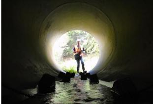
This culvert system was designed and built as part of the 'Transit' ALPURT B1 Project in the mid to late 1990's. The culvert inlet has a simple standard headwall, and there is fish passage through the culvert (simple wooden baffle blocks that were designed and installed prior to the release of any NZ guidance documents on fish passage design). A copy of the relevant engineering layout plan can be seen here: 03328.TIF
