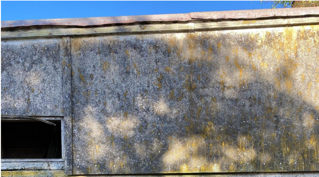
Figure 5.11: Shed with fibre cement cladding.
