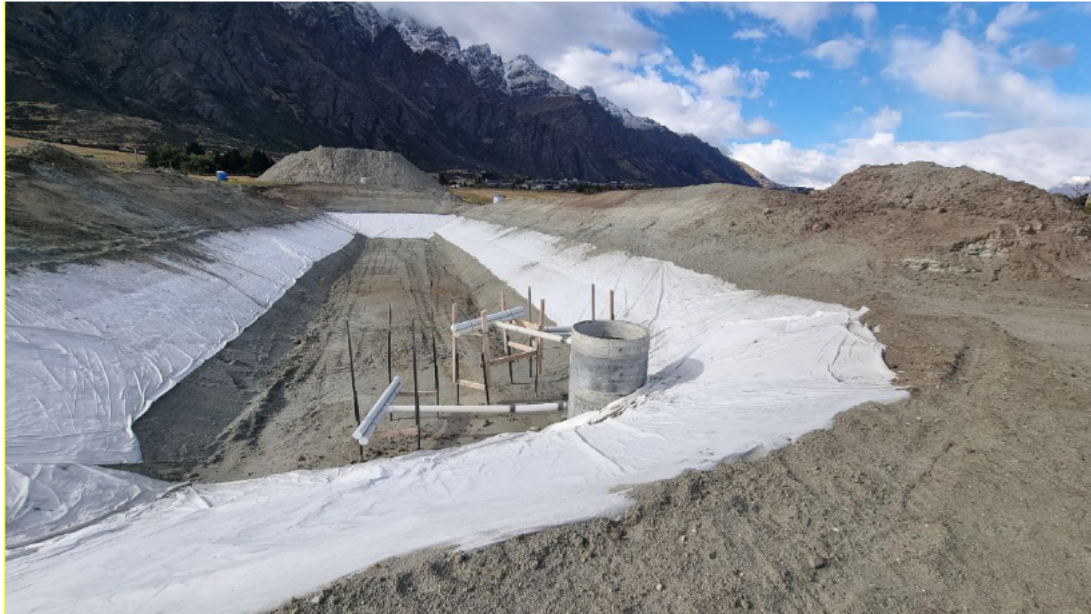
Figure 6-4: Sediment Retention Pond outlet example
