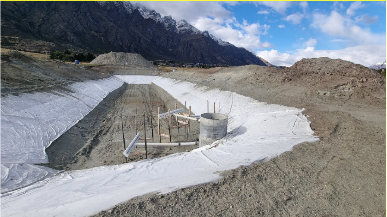
Figure 6-5: Sediment Retention Pond outlet example
