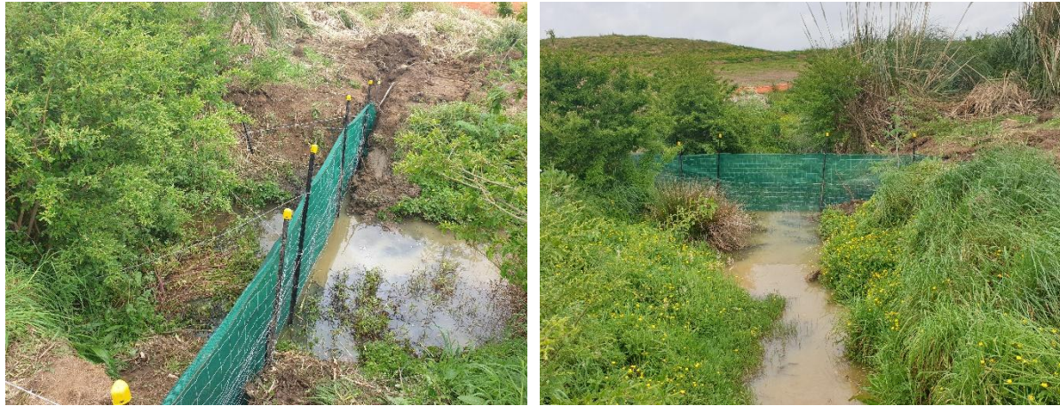
Photo 1 and 2. Photo examples of fish exclusion barriers
