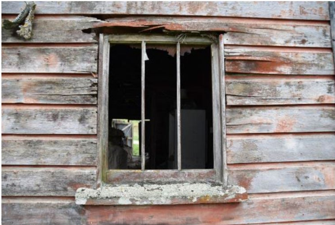
Photo 22 One of the three-light mullion windows at ground floor level to the south elevation (with remaining piece of pressed pattern glass).
