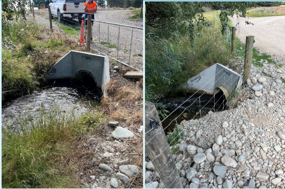
Photos showing upstream (left) and downstream (right) of box culvert at Bendrose Stream crossing.
