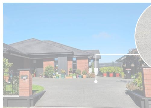
Exposed aggregate concrete with 4% black oxide
