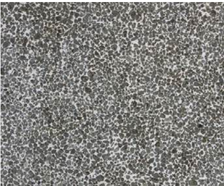
A4 Exposed concrete
