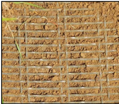
Section of the skirt uncovered for a fence audit.
