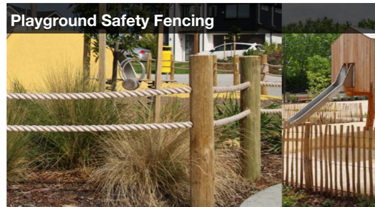
Low soft timber fencing that offers a safety barrier between the play area and nearby roads and driveways with coming and going vehicles. Aesthetic to be non-obtrusive and in keeping with the overall Surf Park.
