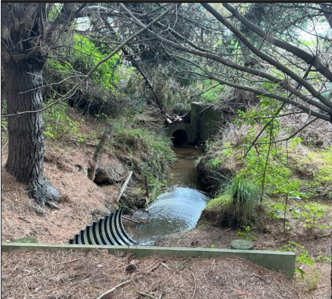
Figure 9. Standing on the middle culvert between SH 59 and driveway.
