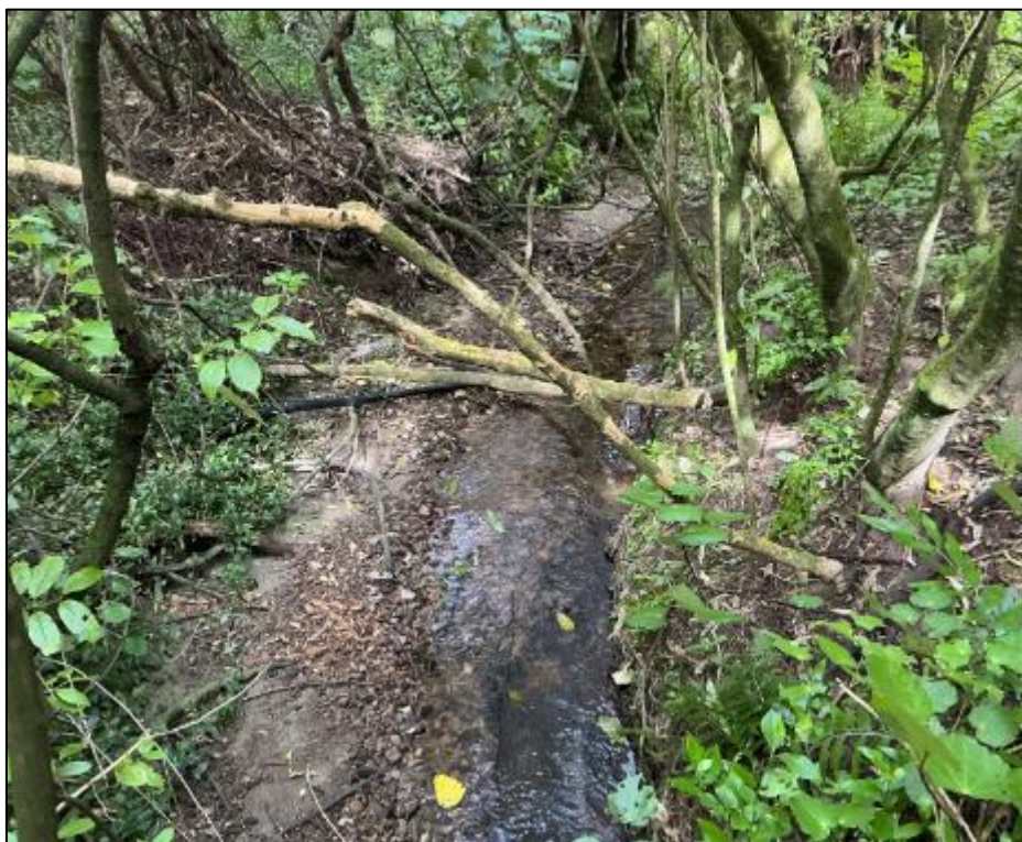
Figure 13. Typical stream bed at the lower end of the proposed culvert pipe to facilitate the roundabout.
