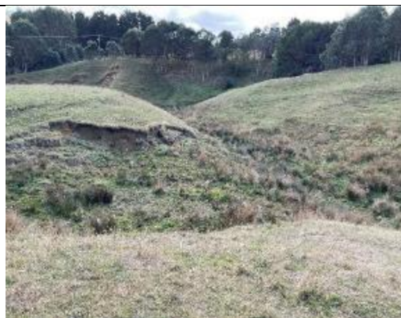
Northern western gully down stream to northern arm (#51-52)
