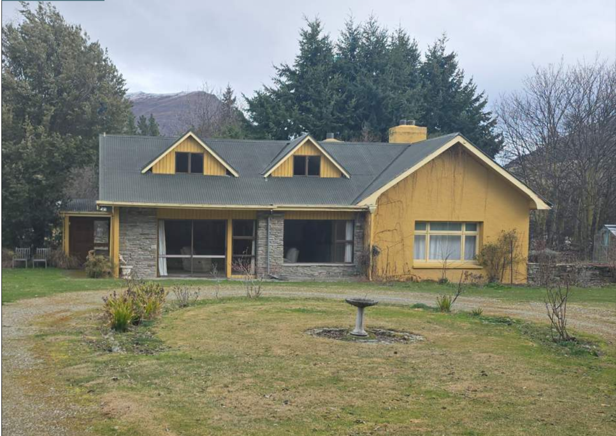
Residential dwelling (Area 1)
