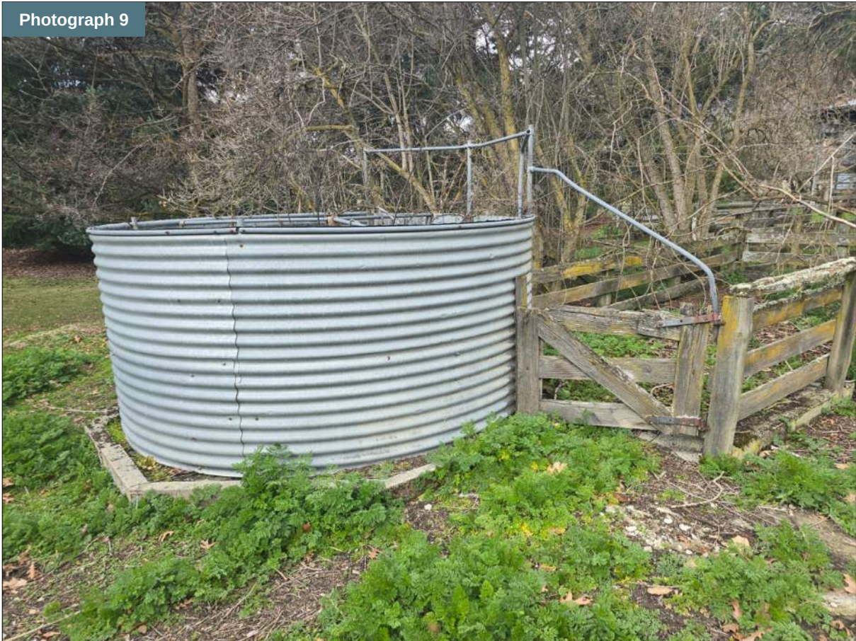
Sheep spray chamber and adjacent stock pens (Area 1)
