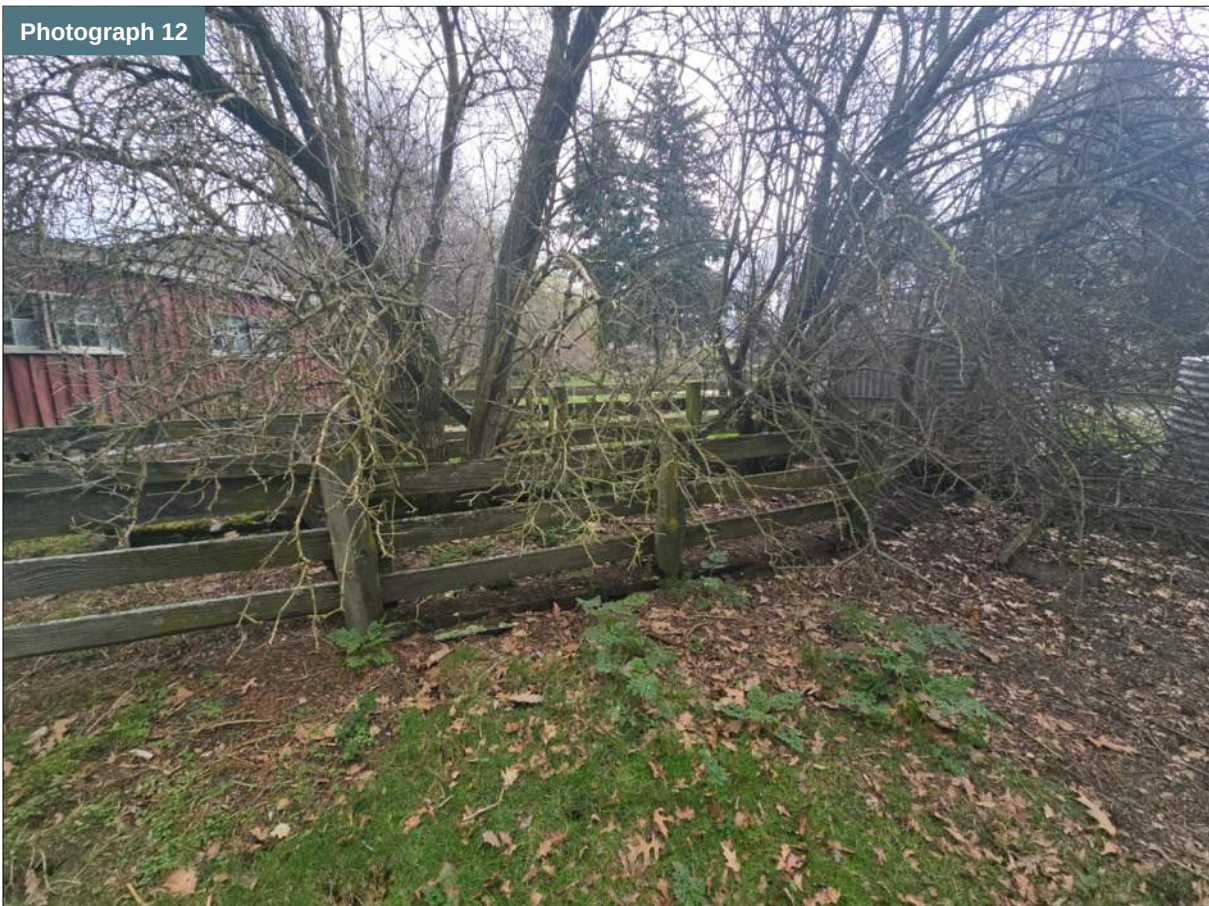
Stock races leading to/from the spray chamber (Area 1)
