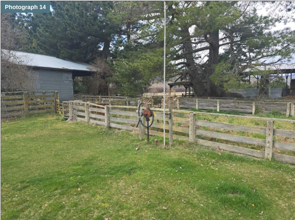
Area of the underground storage tank, with filling points and vent infrastructure visible. Stock holding pens beyond. (Area 1)
