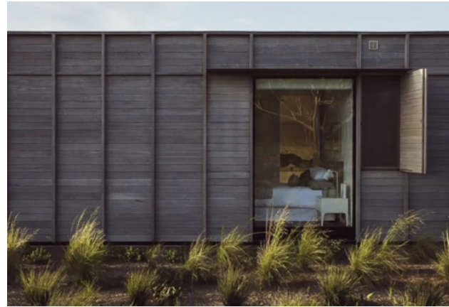
Timber weatherboards with raised batten detail
